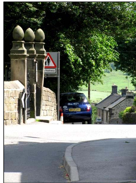
P7.6 Bradford Lane roofs are below eye level
