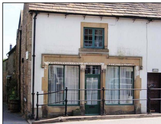
P4.1 Former shop front on Church Street
