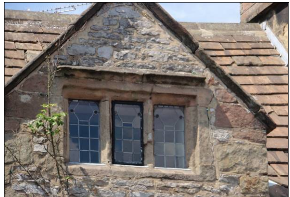
P5.5 Seventeenth century window the Old Hall
