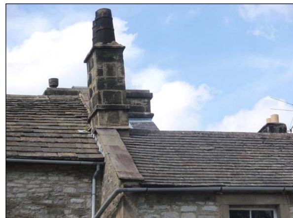
P6.4 A mixture of roof materials, stone slate, clay tile and blue slate, just visible
