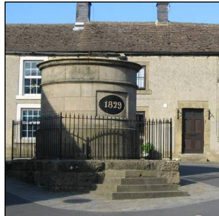
P5.13 The Conduit Head, Fountain Square
