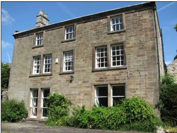
P6.2 The former vicarage has a gritstone façade, other elevations are limestone rubble
