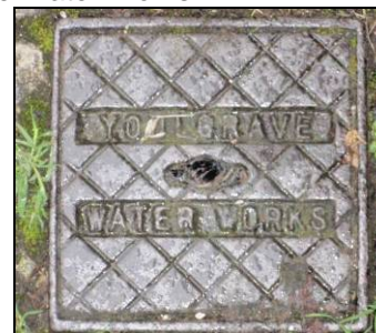
P6.13 Youlgrave Water Works stop tap cover
