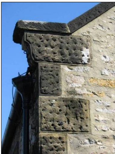
P6.6 Quoins with picked tooled finish and margin detail
