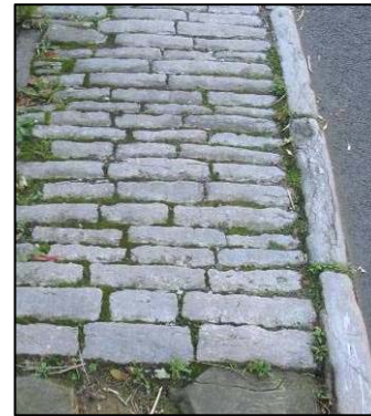
P6.12 Limestone setts at Coldwell End
