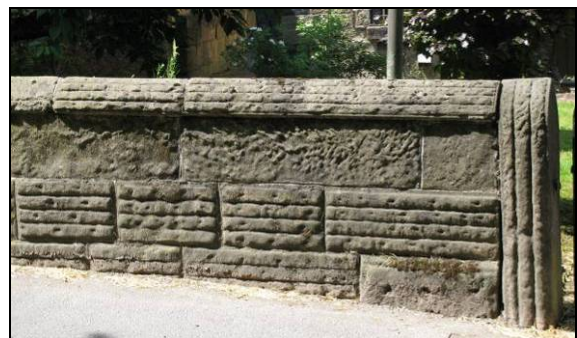
P6.9 Boundary wall to Linden House
