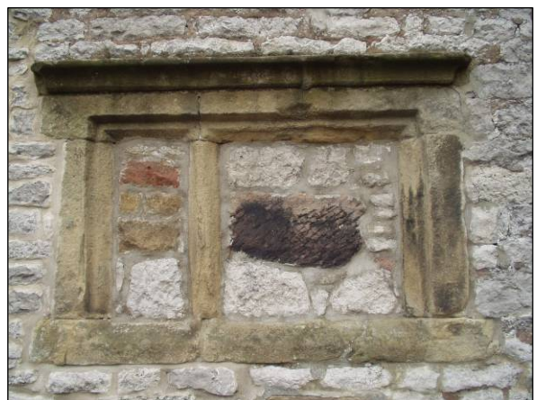
P5.6 Blocked seventeenth century window, Fountain View Cottage
