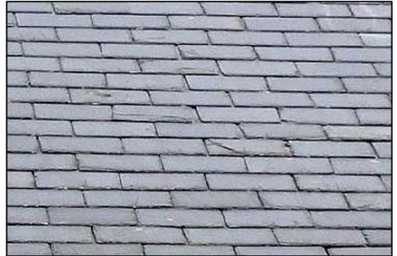
P66 Welsh slate roof
