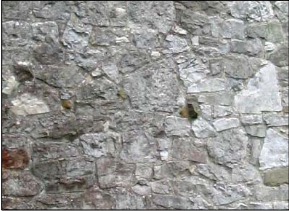
P61 Coursed + uncoursed rubble limestone walls
