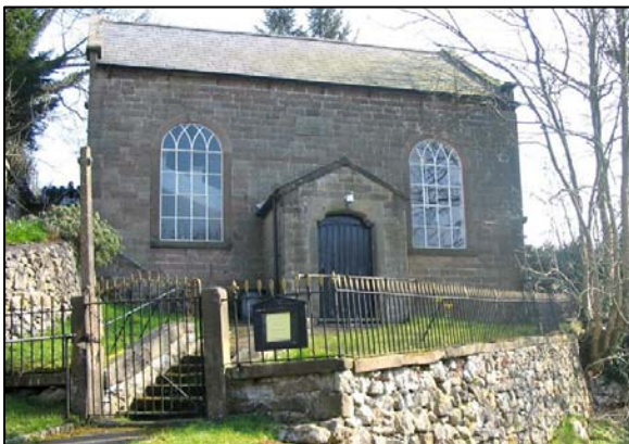
P48 Parwich Methodist Church
