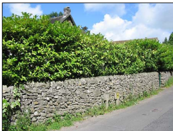
P71 Boundary wall and hedge to Poolcroft
