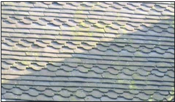
P62 Fishscale clay roof tiles
