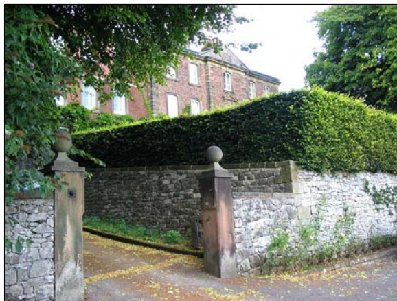
P75 Boundary walls to Parwich Hall
