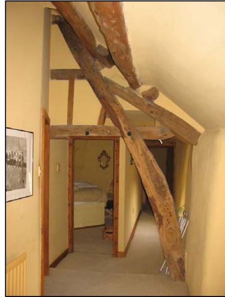
P37 Cruck beams inside Shaw Lane House
