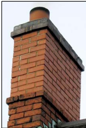
P64 Red brick chimney stack
