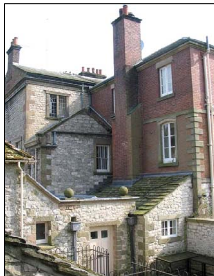
P54 Parwich Hall - red brick & limestone
