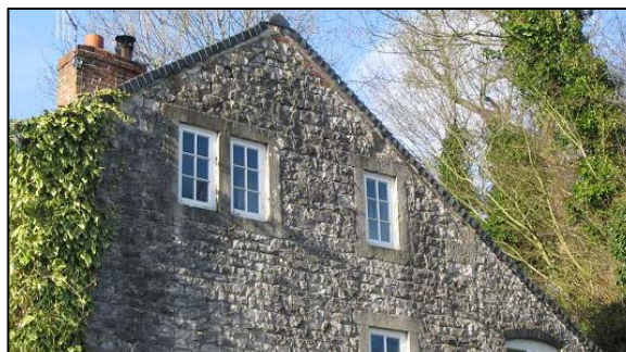
P45 Ridge tiles along eaves at Rose Cottage
