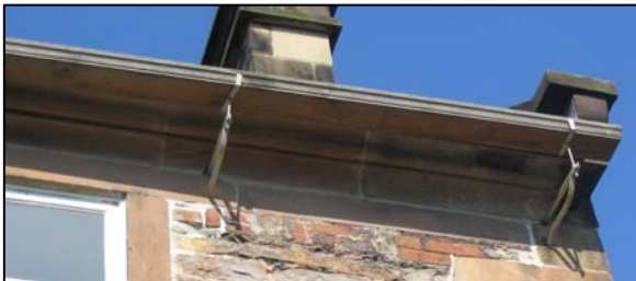
P51 Timber box gutters
