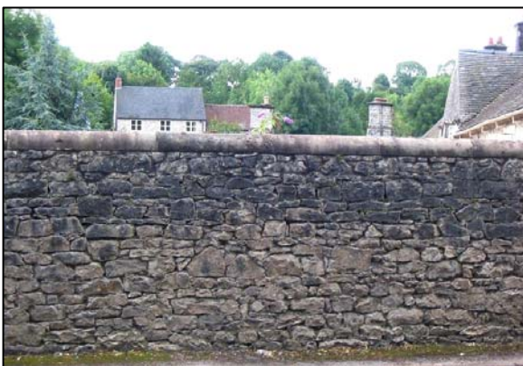
P76 High stone boundary wall to stables
