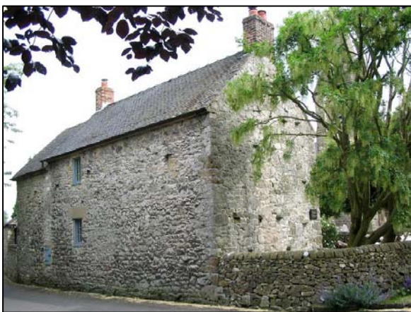
P103 Enclosed feel at entrance to Church Walk
