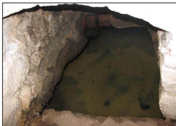
P46 Well in basement at Fernlea
