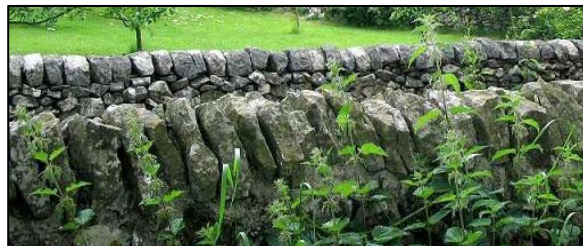
P57 Rubble limestone boundary walls
