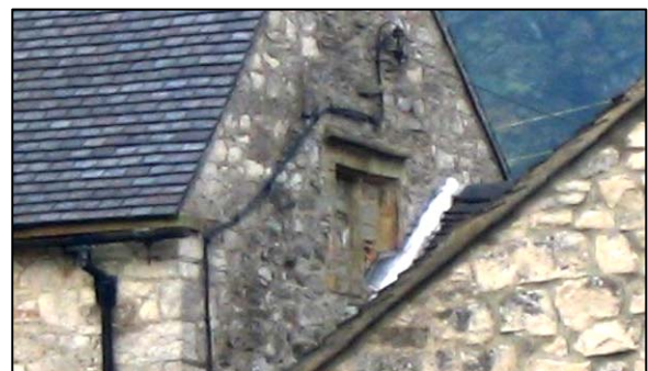
P33 Nethergreen Farm - blocked C17th window
