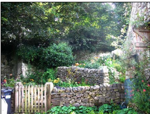
P74 Retaining wall + trees above Rookery House
