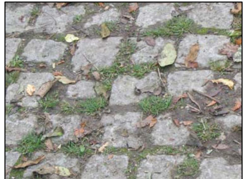
P68 Limestone setts by the shop
