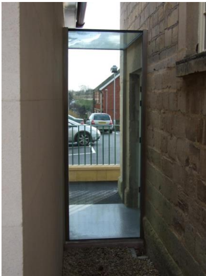
33 (left) A modern glazed link between two buildings. The minimum framing to the glass walls and roof allows maximum transparency and makes the link very unobtrusive. 34 (right) A more traditionally detailed, glazed link built against a high stone wall connecting two buildings.
