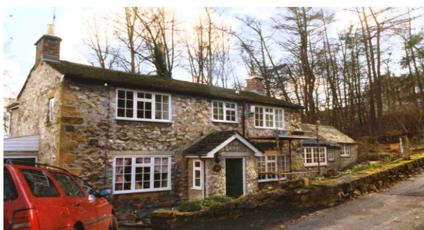
5 (left) BEFORE: a 19th century cottage in Bakewell radically altered by modernisation in the 1970s. (The only clue to the original window openings was a surviving stone sill to the ground floor window on the left hand side.)
