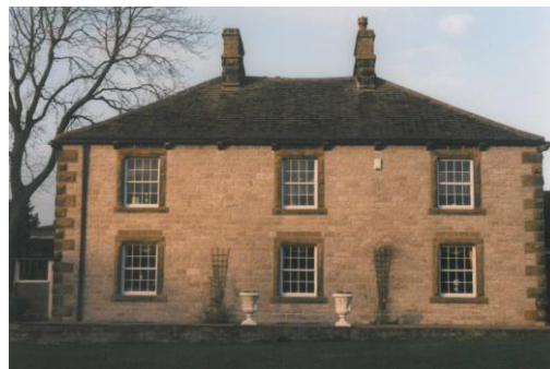
7 (left) BEFORE: modern, unsubdivided sashes in this early 19th century house near Foolow. (Tape has been added to one window to simulate the subdivision proposed.)
