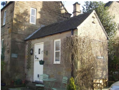
32 (left) A modest, single storey side extension taking its cue in terms of design and materials from the main building.
