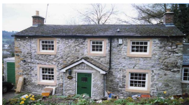
5 (left) BEFORE: a 19th century cottage in Bakewell radically altered by modernisation in the 1970s. (The only clue to the original window openings was a surviving stone sill to the ground floor window on the left hand side.)
