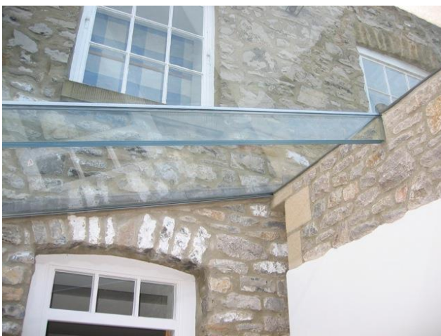
36 This glazed link allowed extension to historic cressbrook mill without harm to the buildings integrity.
