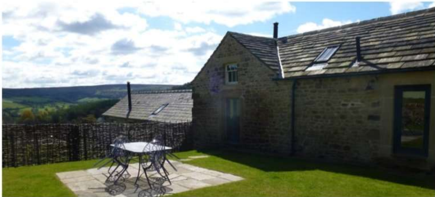
COMPLETED REAR TERRACE
