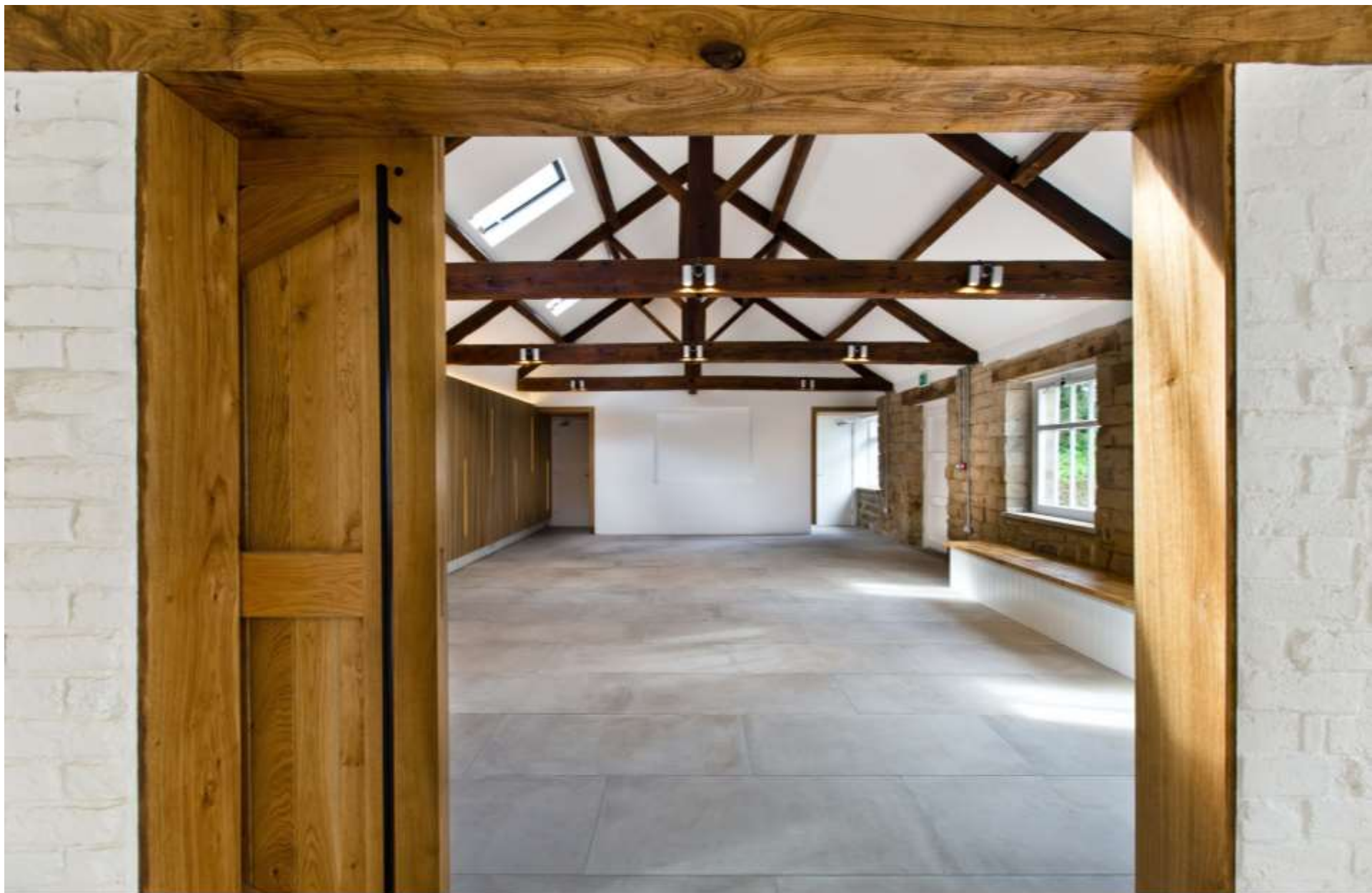
Chatsworth Learning Centre Photo 03 View through opening showing sliding door 16 May 2018
