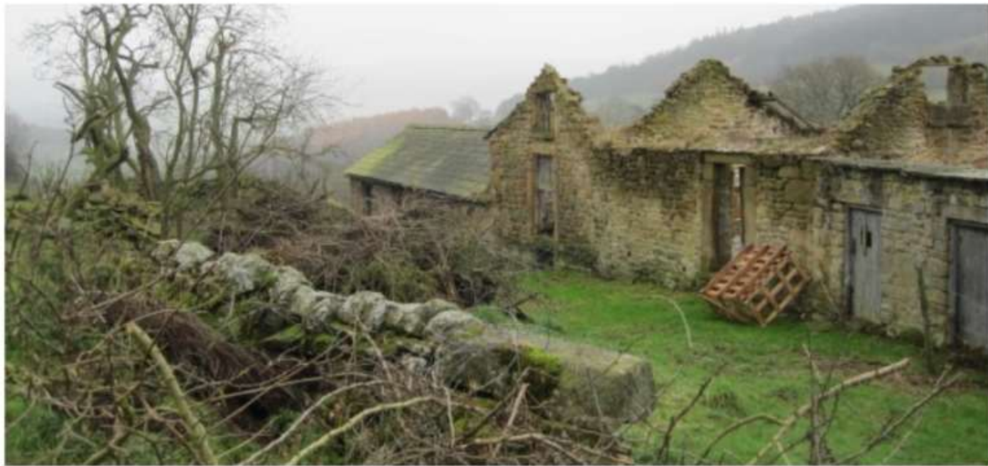
EXISTING REAR TERRACE
