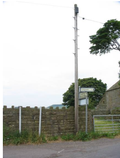
P43 A cluster of signs and posts at the entrance to the hamlet from the Strines direction
