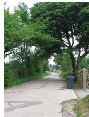
P18 Concrete track at Town End looking towards Well Bank
