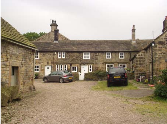
P7 Courtyard arrangement at Well Bank Farm
