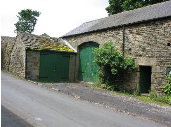
P6 Barn on northern side of road, with openings facing south
