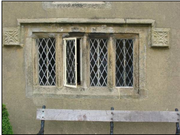
P14 Double chamfered mullion window with hoodmould
