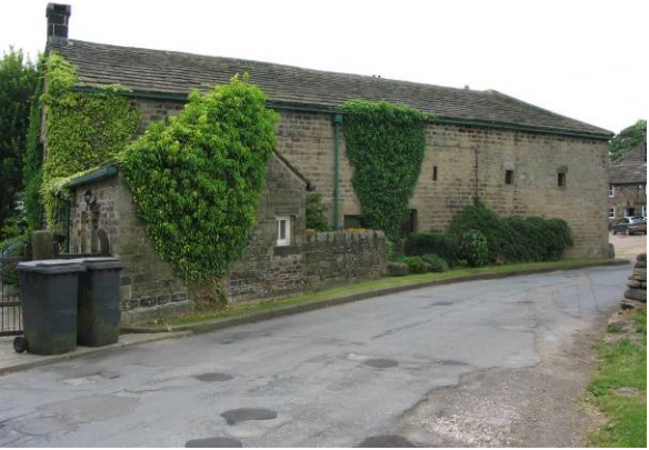
P8 Barn at Well Bank Farm at the east end of the hamlet
