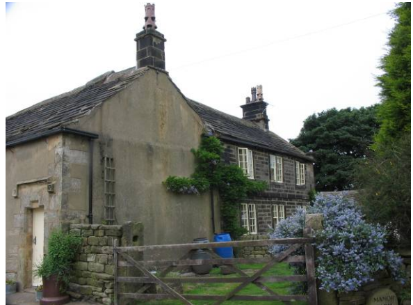
P13 Ashlar chimneys at Manor Farm
