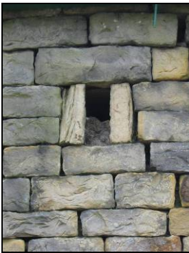
P10 Coursed gritstone barn wall with a ventilation slot
