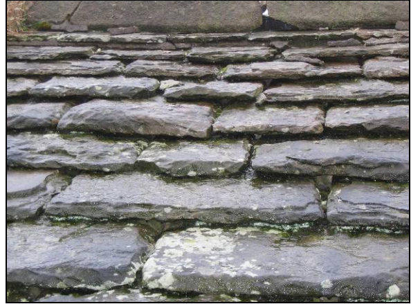
P12 Gritstone roof with stone ridge
