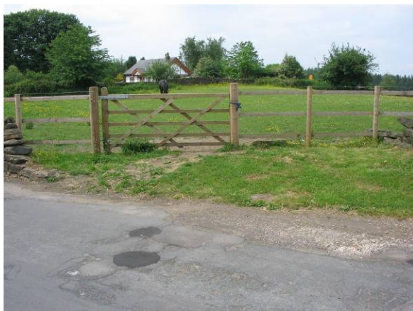
P42 This section of wall is missing creating an open feel
