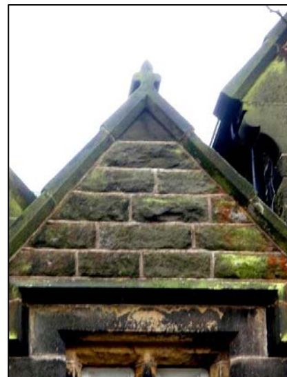
P14 Former Vicarage; vertically grooved chimney stack; fleur-de-lys finial
