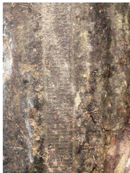
P20 Horizontally tooled vertical band to gate pier
