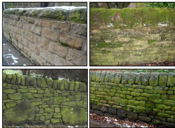
P19 Boundary walls
