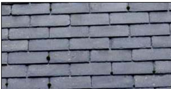
P16 Welsh slate roof
