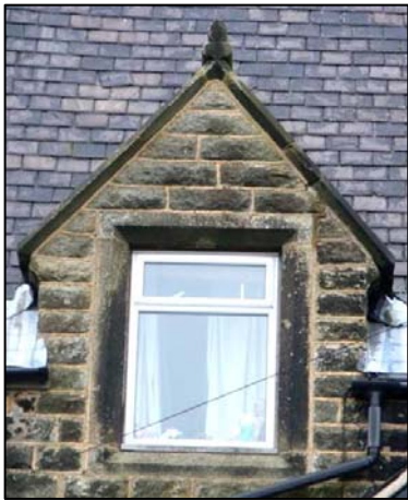
P13 The Old School House; four diagonally set chimney stacks; fleur-de-lys finial
