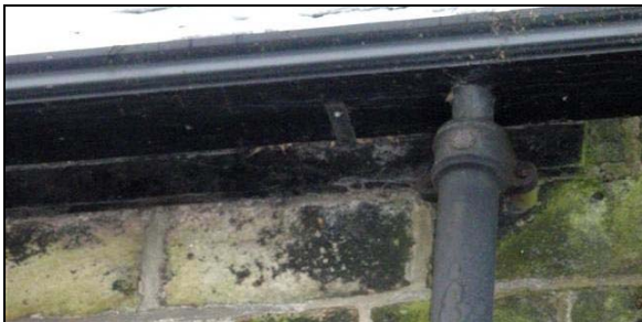
P17 Timber gutter + cast-iron downpipe
