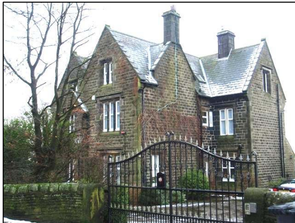
P2 Former Vicarage
