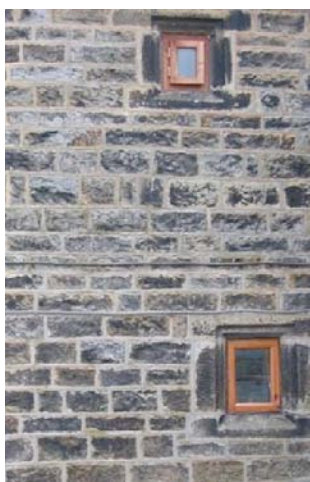
P.5.1. Fire Windows at the property east of Langsett House
