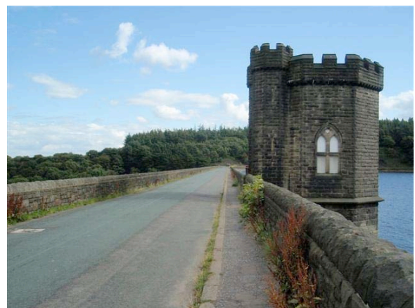
P.10.4. View of the Valve Tower
