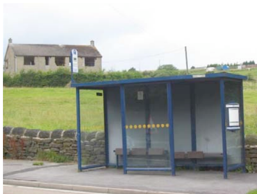
P.11.7. Bus Shelter by the A616
