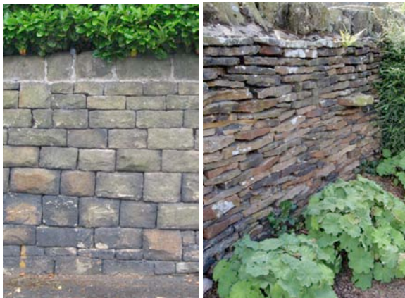
P.6.5. Left: block stone wall with half round copings
