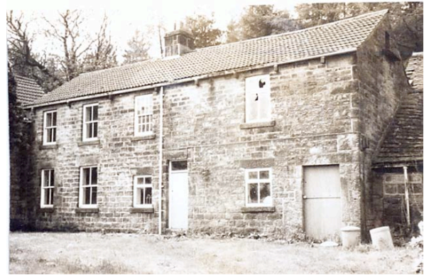
P.3.4. The Dairy at Langsett House, prior to conversion.
