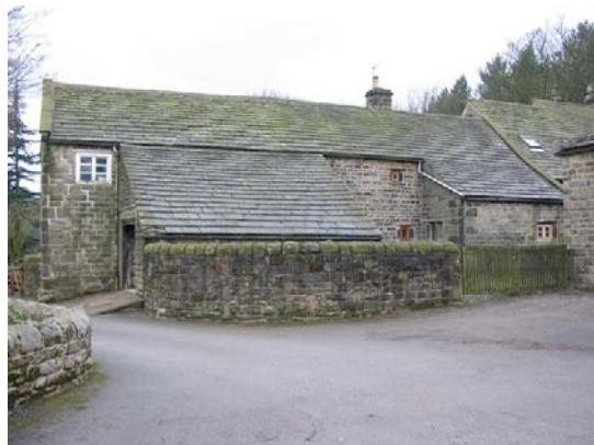
P.7.4. Rear of Langsett Farm House
