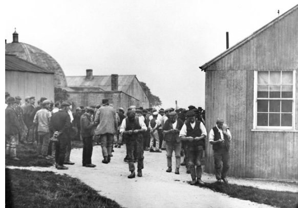
P.3.3. The Metal Prefabricated Buildings in Langsett © Hilary Ambrose
