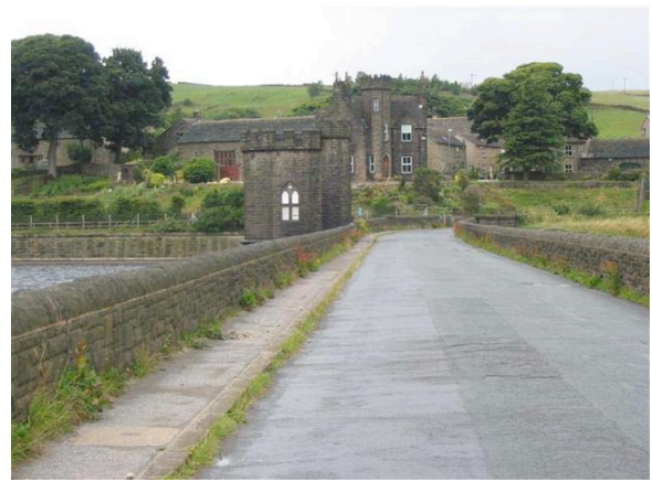
P.10.2. View of the Valve Tower in context with the settlement.
