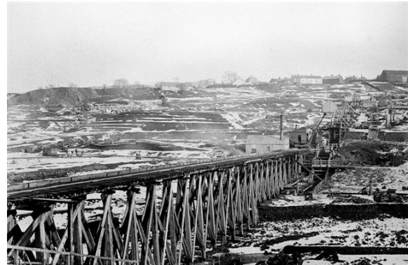
P.3.2 . Constructing Langsett Reservoir © Hilary Ambrose
