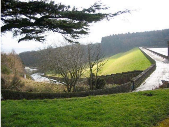
P.9.3. The road over the dam to Cliff Wood.
