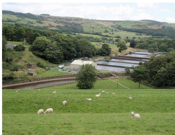
P.9.2. Water Treatment Works to the south-east
