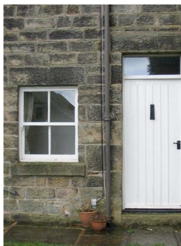
P.5.4. Sash window at the former dairy, Langsett House
