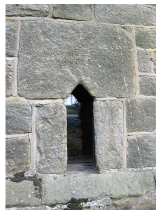
P.6.3. Ventilation slit, Langsett Barn
