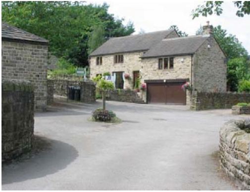
P.7.6. Barnside, part of the Water's Edge
