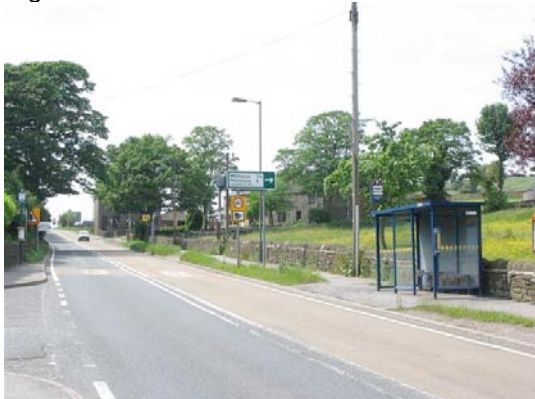
P.11.5. The section of A616 within the Conservation Area.
