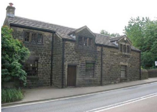
P.5.5. School House Cottage
