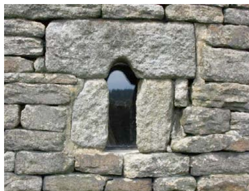
P.6.2. Ventilation slit within the barn north of the Lodge
