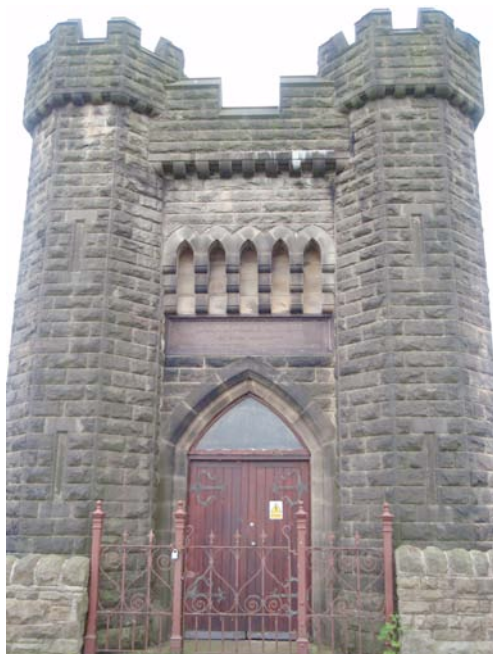
P.10.1. Front Façade of the Valve House.
