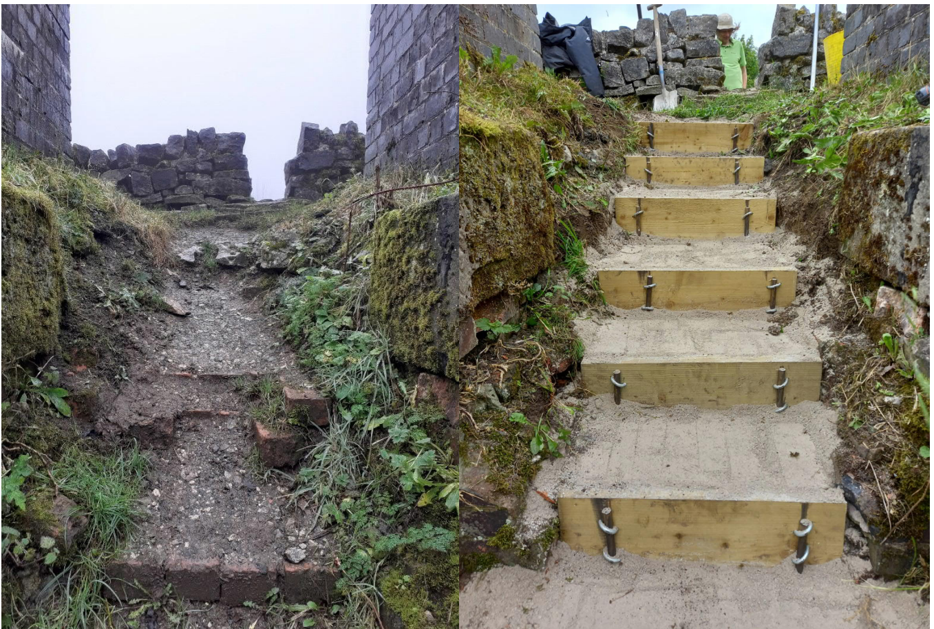
Step repairs before and after
