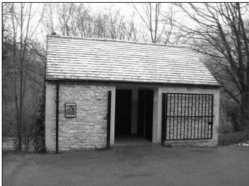
External information panel at White Lodge 'composting toilets'.
