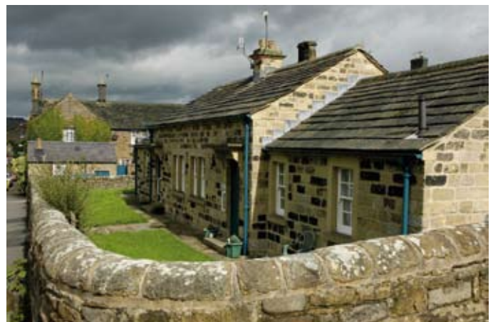
Local needs bungalows, Pilsley: gritstone in the walls have been reused up to five times in the last 250 years
