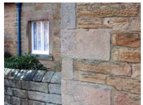
Roughly coursed gritstone walls and quoins, Pilsley
