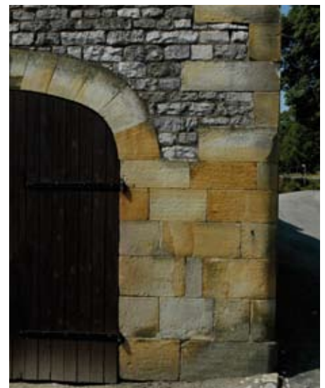
Coursed limestone over ashlar gritstone, Hartington
