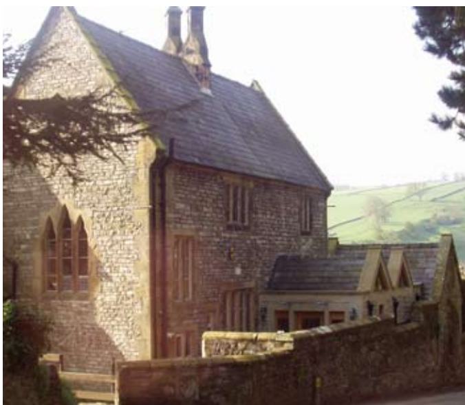
New ground floor extension, Ashford
