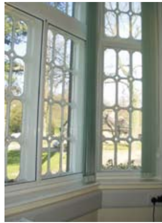
Secondary glazing, Newholme Hospital, Bakewell
