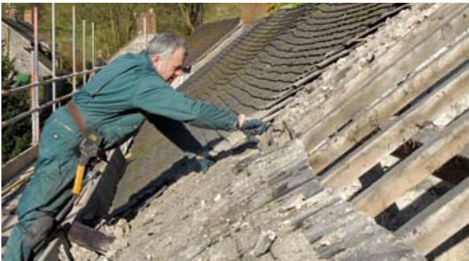
Stripping a blue tile roof prior to reroofing, Parwich
