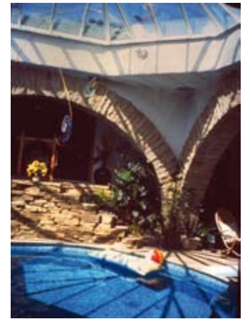
Central space to Underhill, Holme: the underground design gives the building high insulation values
