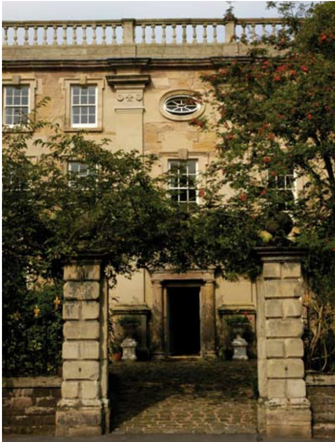
Winster Hall, restoration of entrance courtyard
