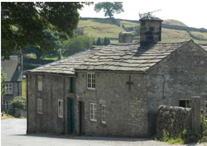
Low eaves, blank gable and ridge stack, to cottage, Hartington
