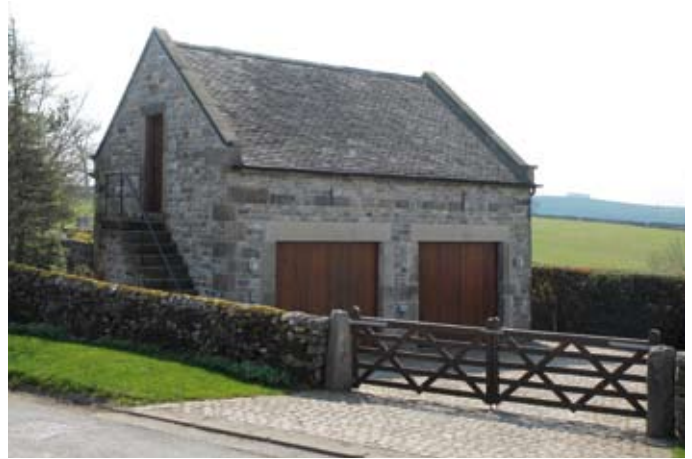
New garage designed as outbuilding, Alstonefield
