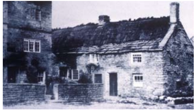
Stone slates at the base of a now demolished cottage with heather thatch roof, Monyash
