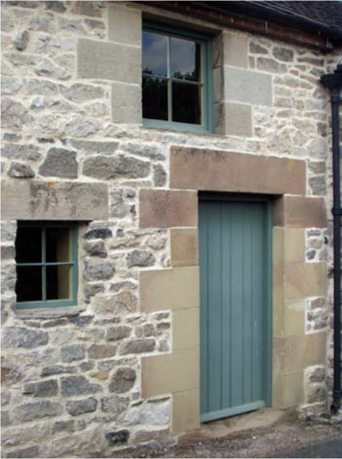
Appropriate, recessive colour to exterior joinery, outbuildings, Parwich
