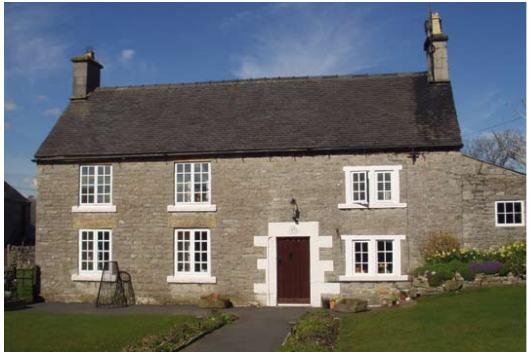
Traditional south facing farmhouse, Alstonefield
