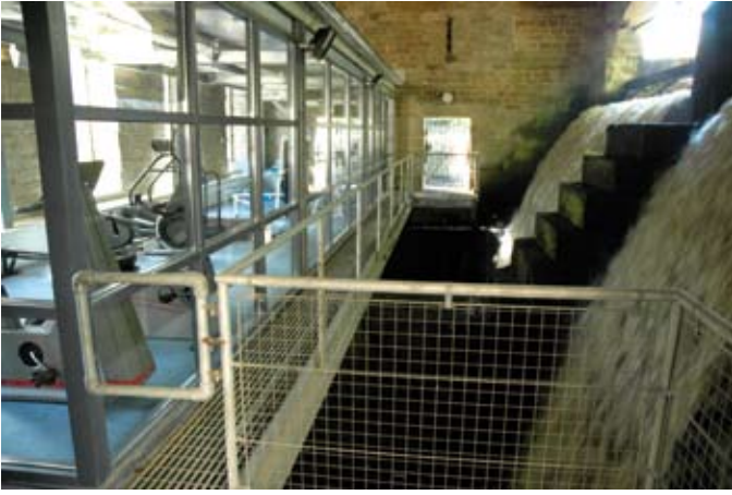
Small gymnasium in part of a listed wheelhouse, Calver Mill
