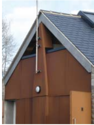
Cor-ten steel cladding, Parsley Hay Visitor Centre
