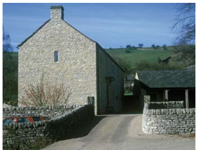
New house in Calver, showing traditional form and gable width
