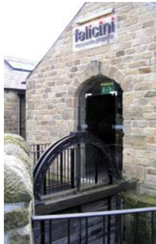
Glazed doorway at a former marble mill, Bakewell
