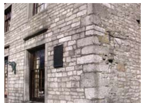
Coursed limestone on the front and rubble limestone on the side. and peculiarly to Monyash, limestone quoins on the corner and limestone surrounds to the openings
