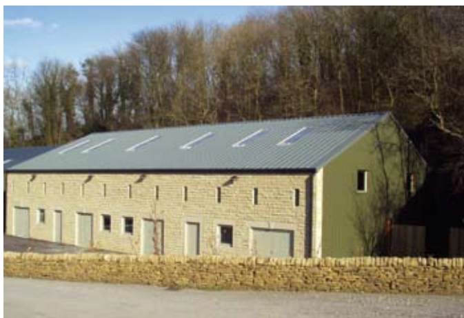
New factory units set into hillside, Bakewell
