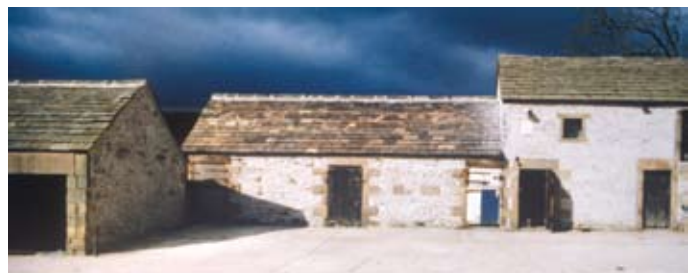
Relaid stone slate roof, Near Middleton by Youlgreave
