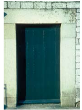
Boarded door with paint finish
