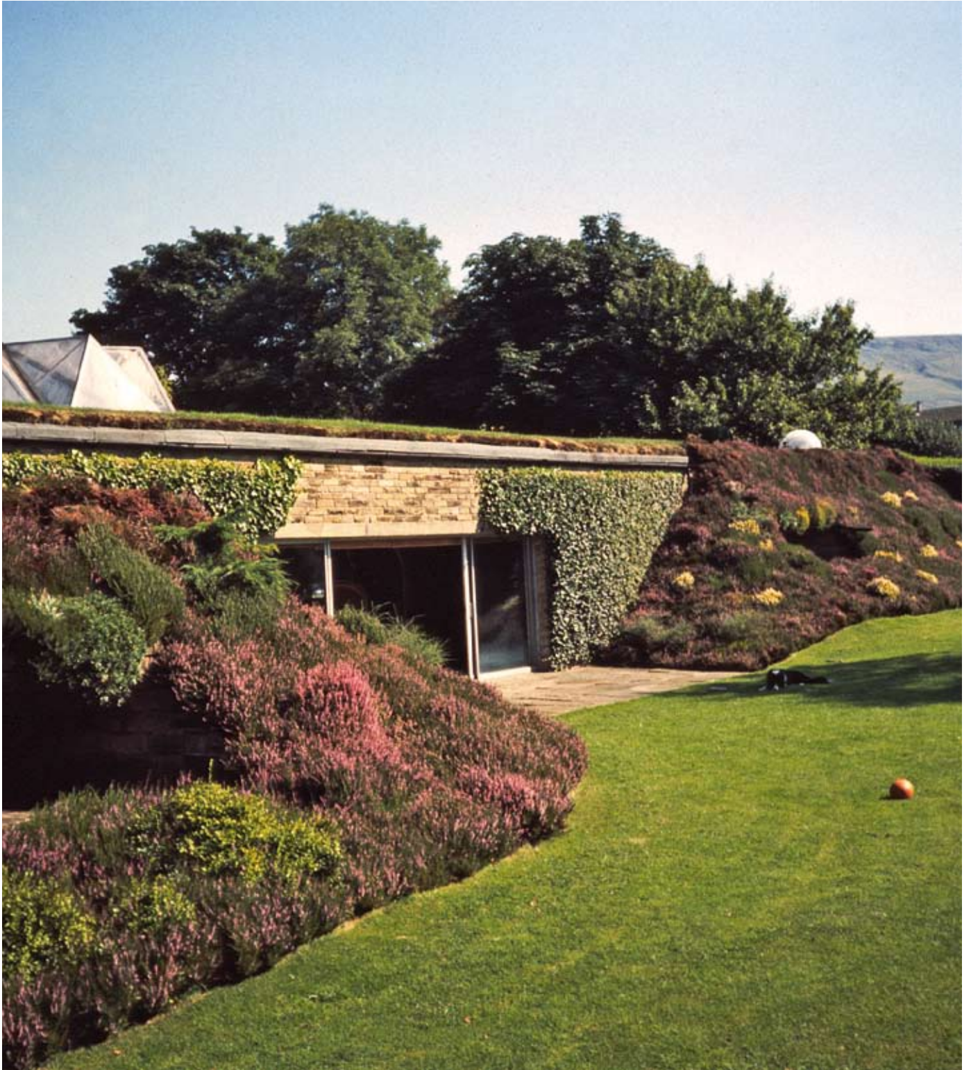
Underhill, underground house at Holme
