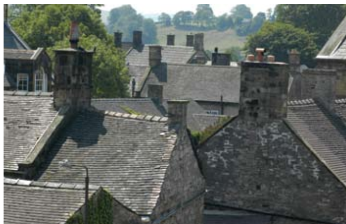
Staffordshire blue clay tiles, Hartington
