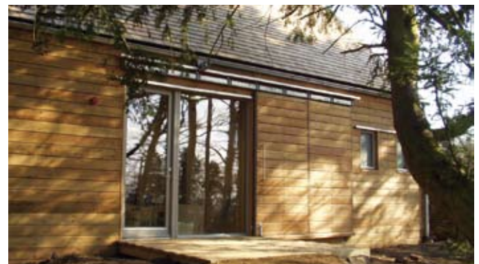
Moorlands Discovery Centre, Longshaw Designed to maximise solar gain and minimise heat loss, with a ground source heat pump to provide heating. The woodland setting makes the use of timber here more appropriate.
