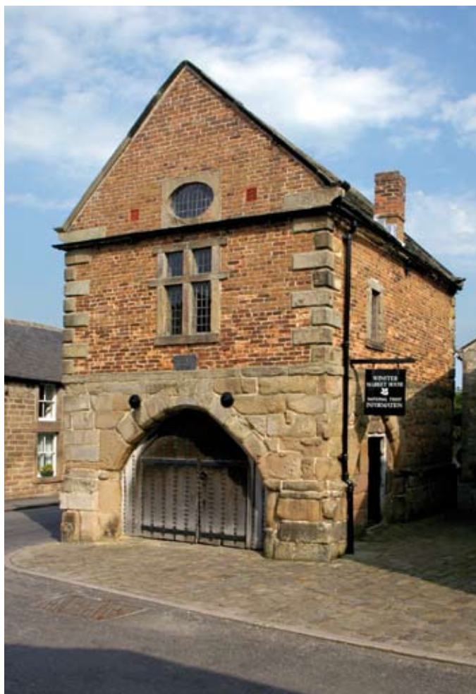
Winster Market hall: a brick first storey above a gritstone base
