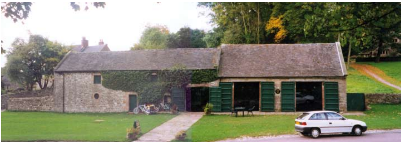
Redundant outbuilding converted to a tea room, Tissington
