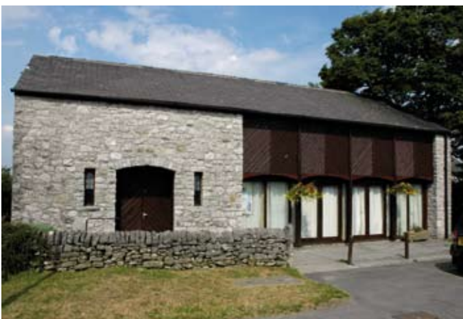
Village Hall, Monyash - form and materials of this self-built hall follow the tradition but detailing is modern
