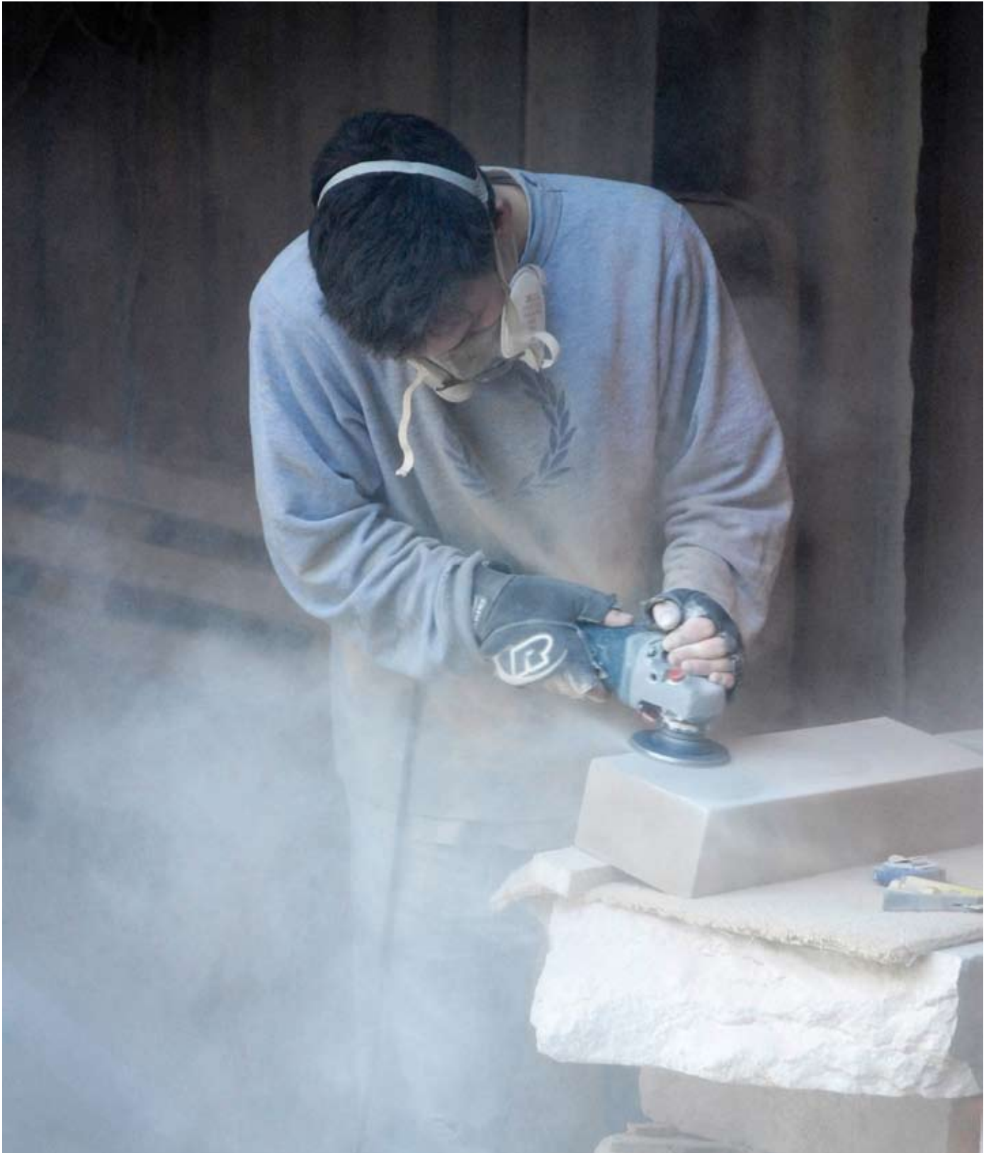
Joe Redfern, apprentice stonemason at R.M.H. Eaton taking a chamfer off a cill
