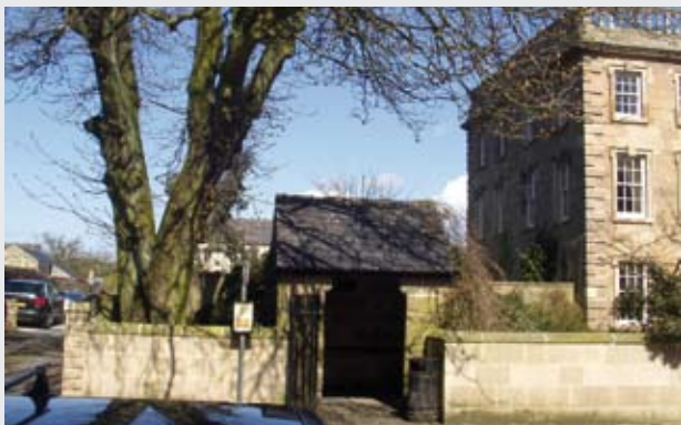
New garden walls and relocated bus shelter help to restore the street frontage
