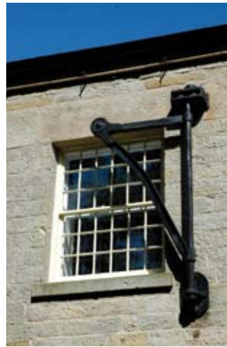
Small paned sash in a former industrial building, Calver
