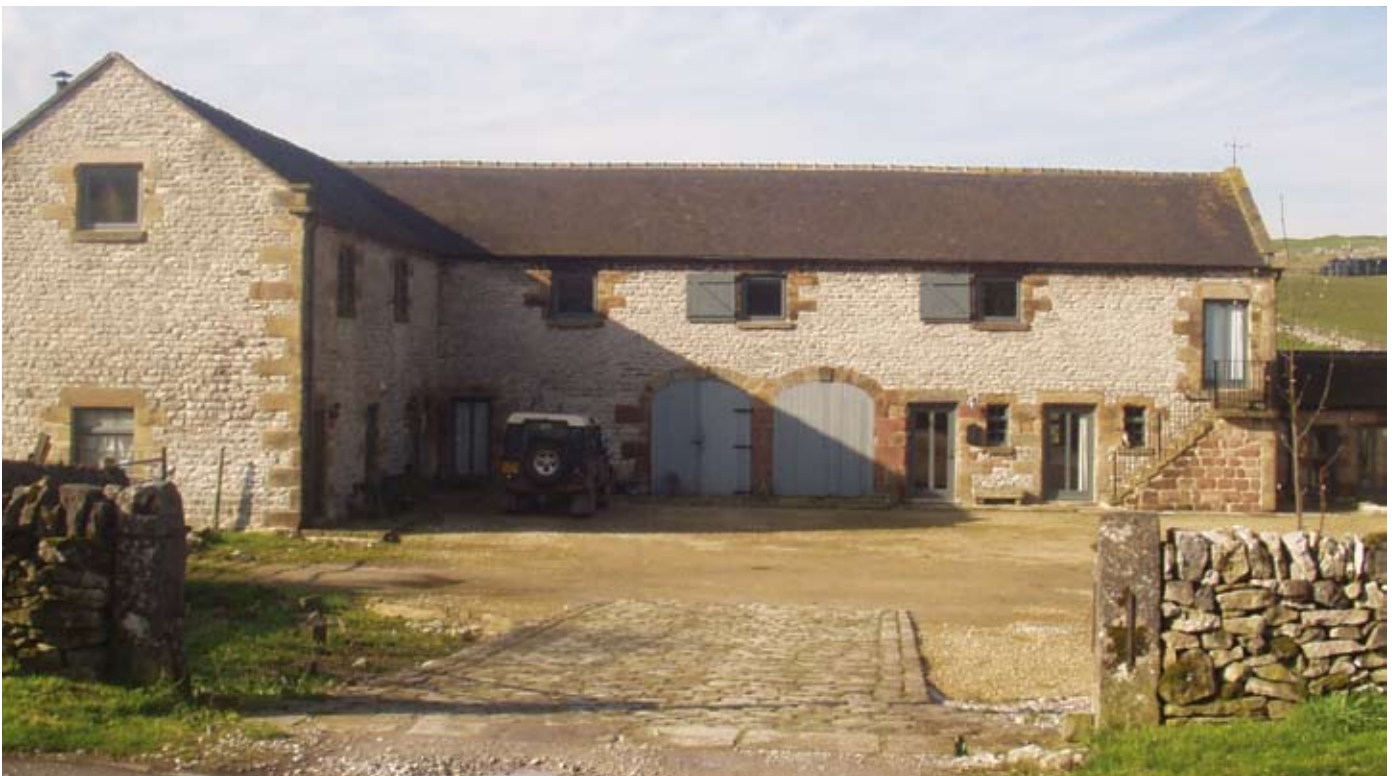
Listed farm outbuilding converted into 2 dwellings, Earl Sterndale (note the unsubdivided courtyard and retention of large ground floor openings for storage)
