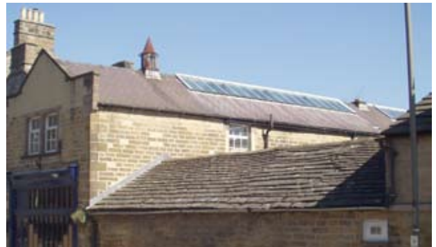
Patent glazing at ridge level on a former workshop, Bakewell
