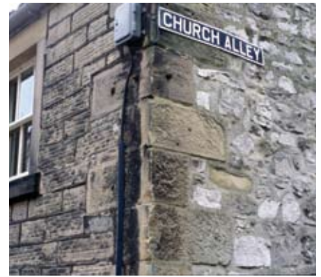
Coursed gritstone on the left meets rubble limestone on the right, Bakewell
