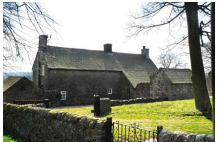
Largely blank rear elevation of a traditional house, Warslow
