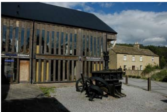
Retention of individual character, Rutland Works, Bakewell
