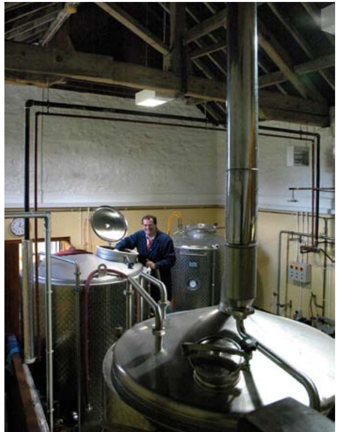
Use of a former barn as a microbrewery, Pilsley
