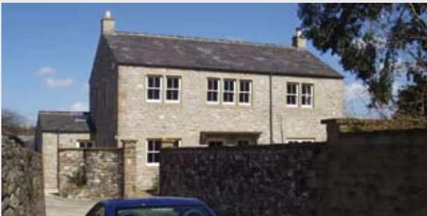
Subsequently refronted with openings reconfigured
