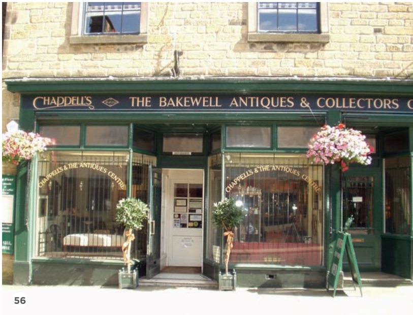
56: Permanent bars fitted inside the window (King Street, Bakewell)
