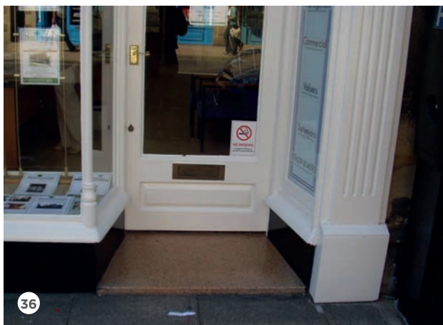
36: Recessed door in C19 shop front
