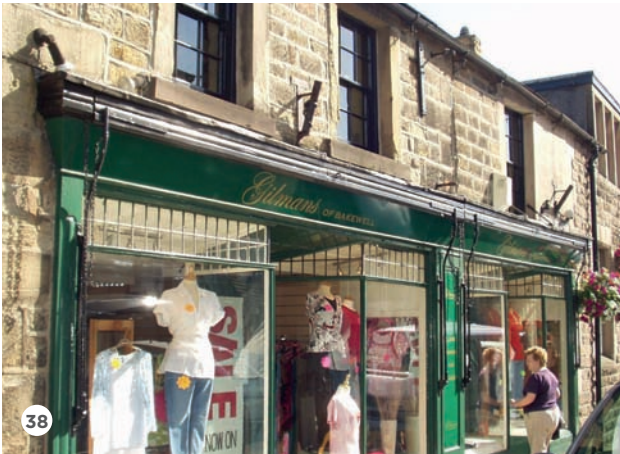
38: Projecting cornice incorporating traditional blind box
