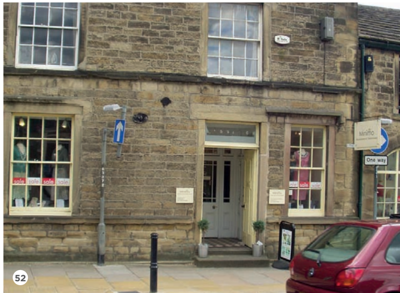
52: Minimal signage - hanging sign and wall-mounted boards
