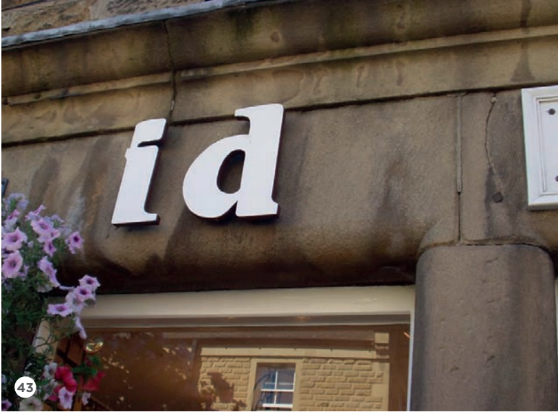
43: Applied letters onto stone fascia (Matlock Street, Bakewell)
