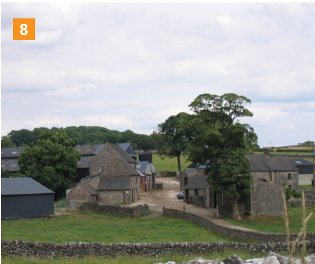
▲ 7. Farmstead set below the moor edge on the High Peak, one of many linear farmsteads occupying a remote and isolated position. It lies amongst fields of piecemeal enclosure, taken in from the moor by the 18th century. Photo © Jen Deadman
