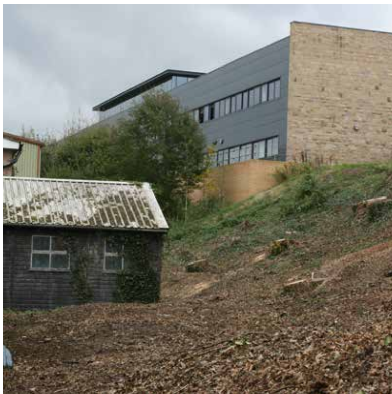
The Repton Sports Facilities site before demolition, from the west looking east along the sandstone bluff
