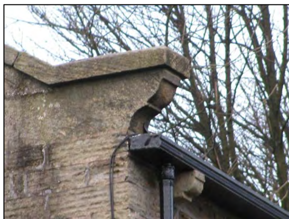
P6.4 Timber gutter on stone corbel support
