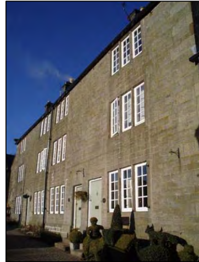
P3.6 Former Workhouse in High Bradfield
