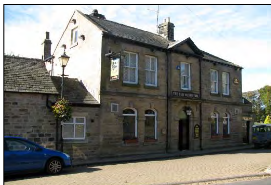
P4.2 The Old Horns Inn, Towngate
