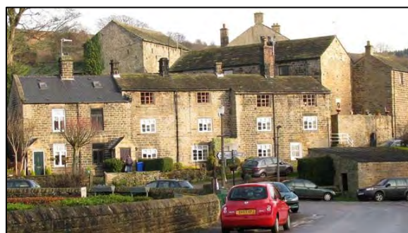
P7.16 Roofs appear one above the other at Burnside Cottages
