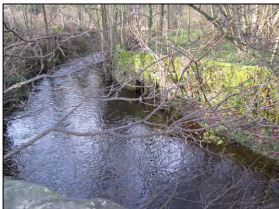
P4.1 Looking down Dale Dike towards the site of the former Corn Mill
