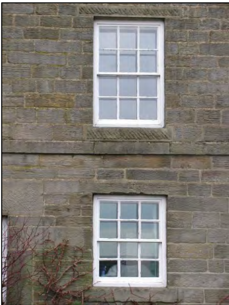
P6.6 Sash Windows at High Bradfield
