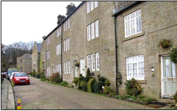
P7.4 Towngate buildings close to the lane edge
