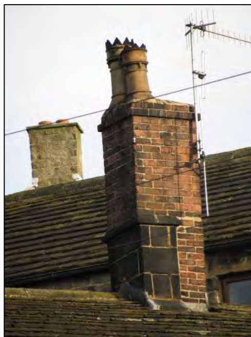
P6.3 An ashlar stack 'smothered' by a red brick chimney
