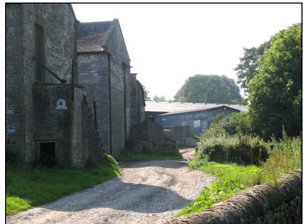
P3.4 Agricultural buildings at Monyash House Farm
