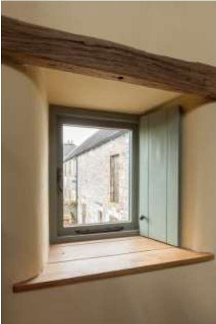
Figure 3 Insulated lime plaster walls conserve the internal appearance of the historic building whilst conserving energy. Home made internal shutters also conserve energy
