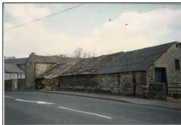
P.3.10. The single storey wing to the Coach-house, Haddonfields, in the 1980s
