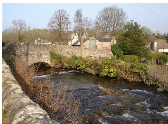
P.2.1. Alport Conservation Area
