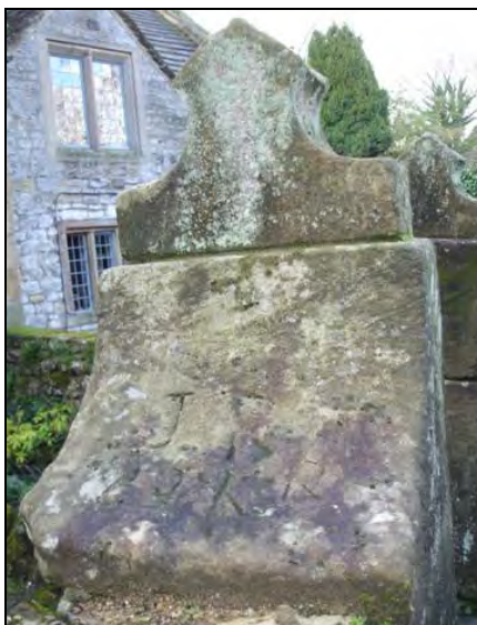
P.3.2. Initials JR incised in the coping to the gate-piers at Monks Hall
