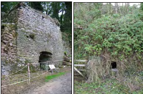
P.4.3. Left: Limekiln immediately east of the corn mill
