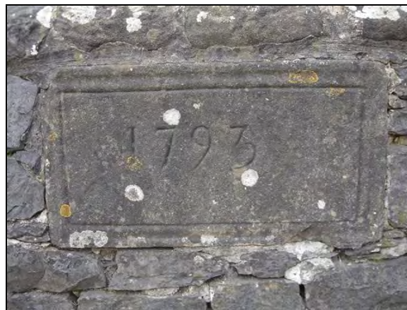
P.3.4. 1793 datestone within the bridge wall
