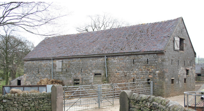
A large combination range, mainly cattle housing with a loft above but with full height crop storage in the end bay marked by the ventilation slits in the right gable end. Photo © Bob Edwards
