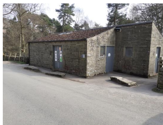
Toilet block at Hollins Bank car park
