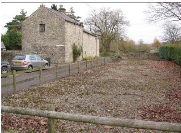
P11.2 Inappropriate fencing on Soft Water Lane (this is temporary)
