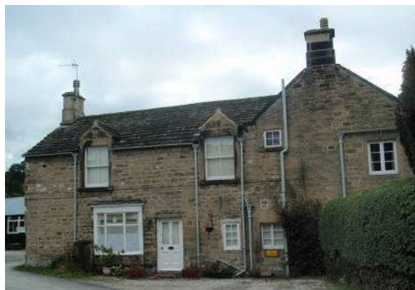
P6.1 cast iron rainwater goods on Bank House
