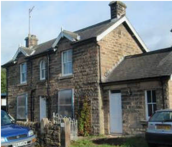
P3.3 Granby Cottage with 'blocked in' post box to single storey extension
