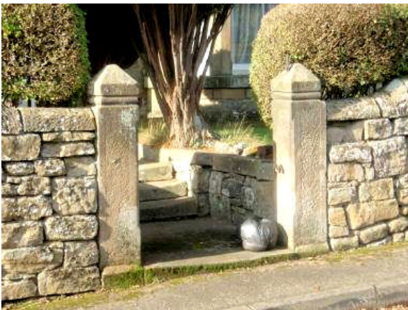
P6.4 Gate posts with framed picked tooling, rolled collars and chamfered points at Fern Bank.
