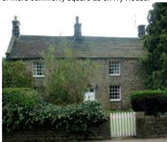
P6.2 square chamfered window dressings on Ivy House
