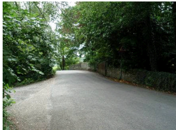
P8.5 Overhanging trees on Wye Bridge
