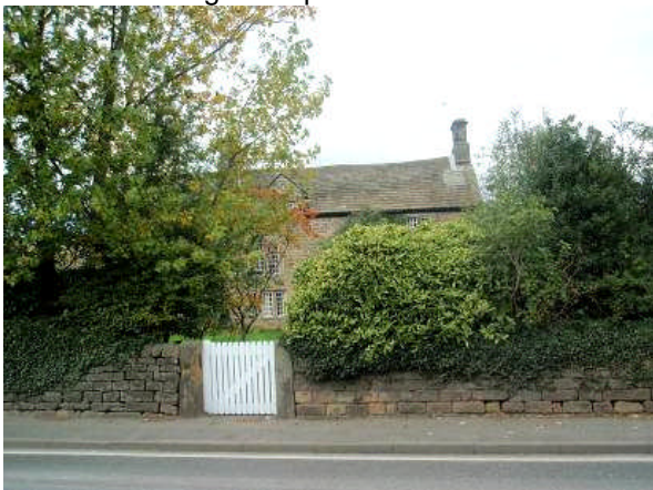
P7.13 Holly House screened by mature shrubs and beech hedging
