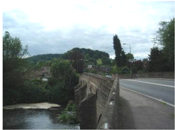
P3.1 Rowsley Bridge
