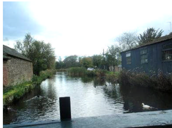
P7.20 View along millrace
