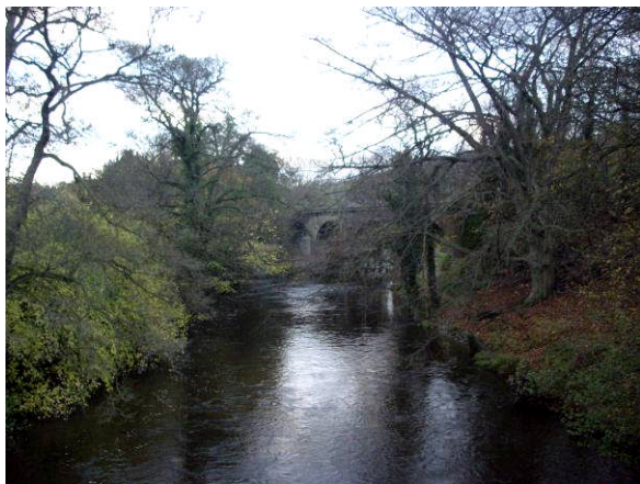
P7.11 View of viaduct from Rowsley Bridge
