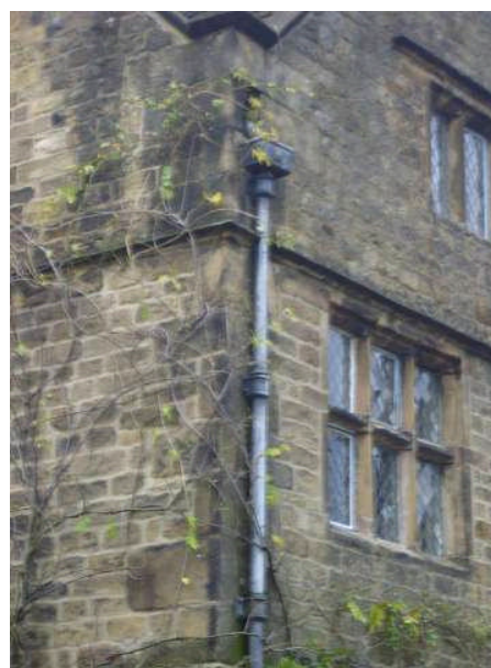
P5.3 Narrow mullioned windows on The Peacock Hotel
