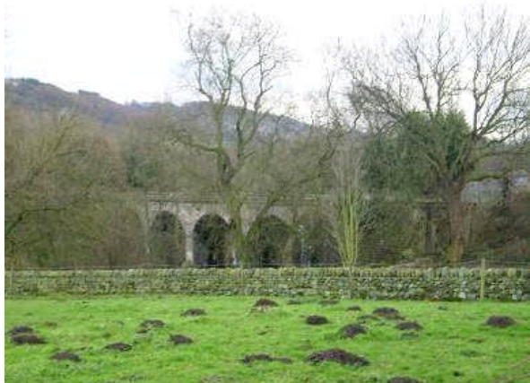
P7.8 View of viaduct from churchyard extension
