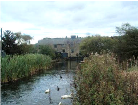
P7.22 View down millrace towards mill
