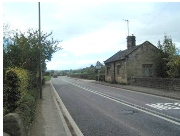
P7.14 View westwards along A6
