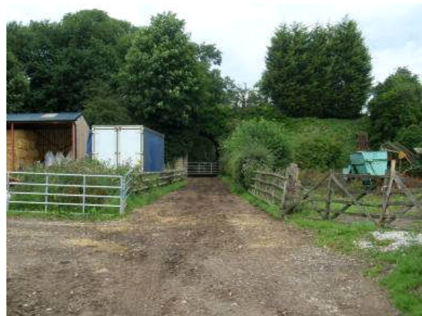
P7.6 Footpath under viaduct arch of Church Lane
