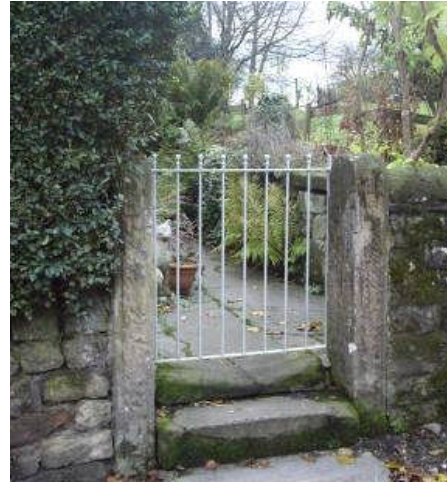
P6.5 Cast iron gate at the Cottage
