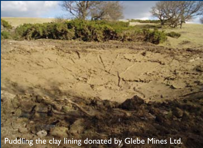
Laying the clay setts. This is a very labour intensive process and makes the pond re-creation very costly. Much of the work has been funded initially by a grant from the Aggregates Levy Sustainability Fund and more recently by Landfill Tax (through the SITA Trust)
