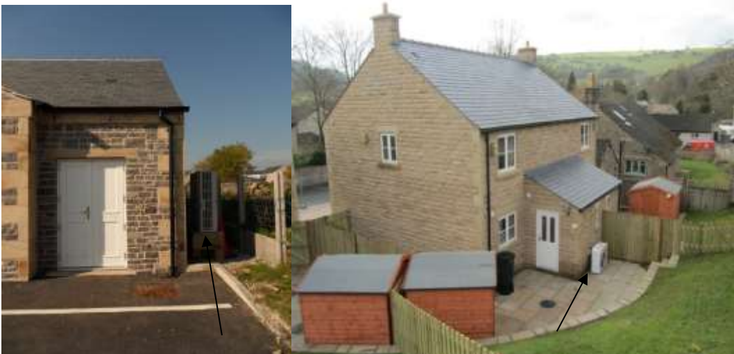
Figure 29. Air source heat pumps at Over Haddon Village Hall and on a new affordable home in Calver
