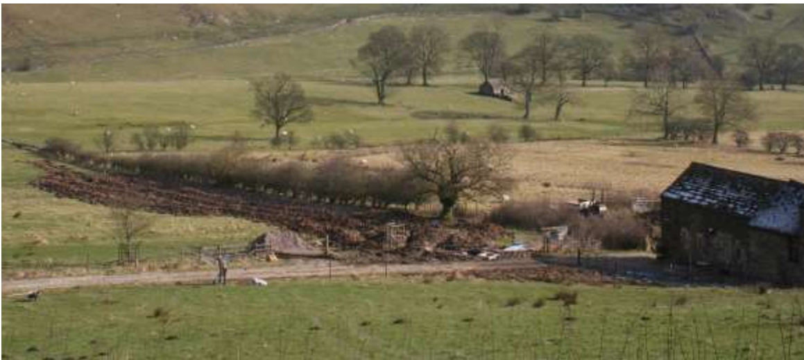
Figure 27. Ground source heat pump excavation
