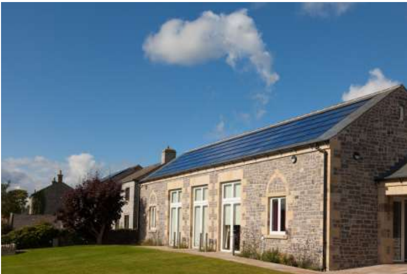
Figure 26. Over Haddon Village Hall
