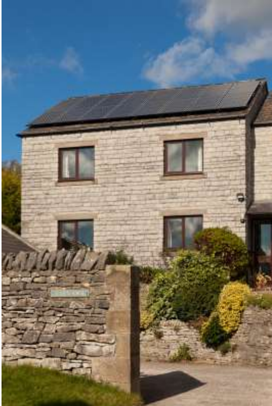
Figure 23. Retrofitted photovoltaics, Over Haddon
