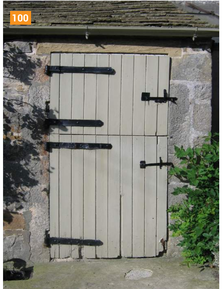
▲ 99. Early 19th century or earlier double doors to a barn with wooden latches and wrought iron hinges. Photo © Bob Edwards
