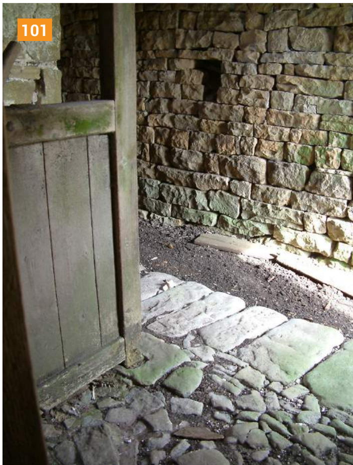
◀ 101. It is common to find slabs used for the walkways and cobbles for the standing areas. Photo © Jen Deadman
