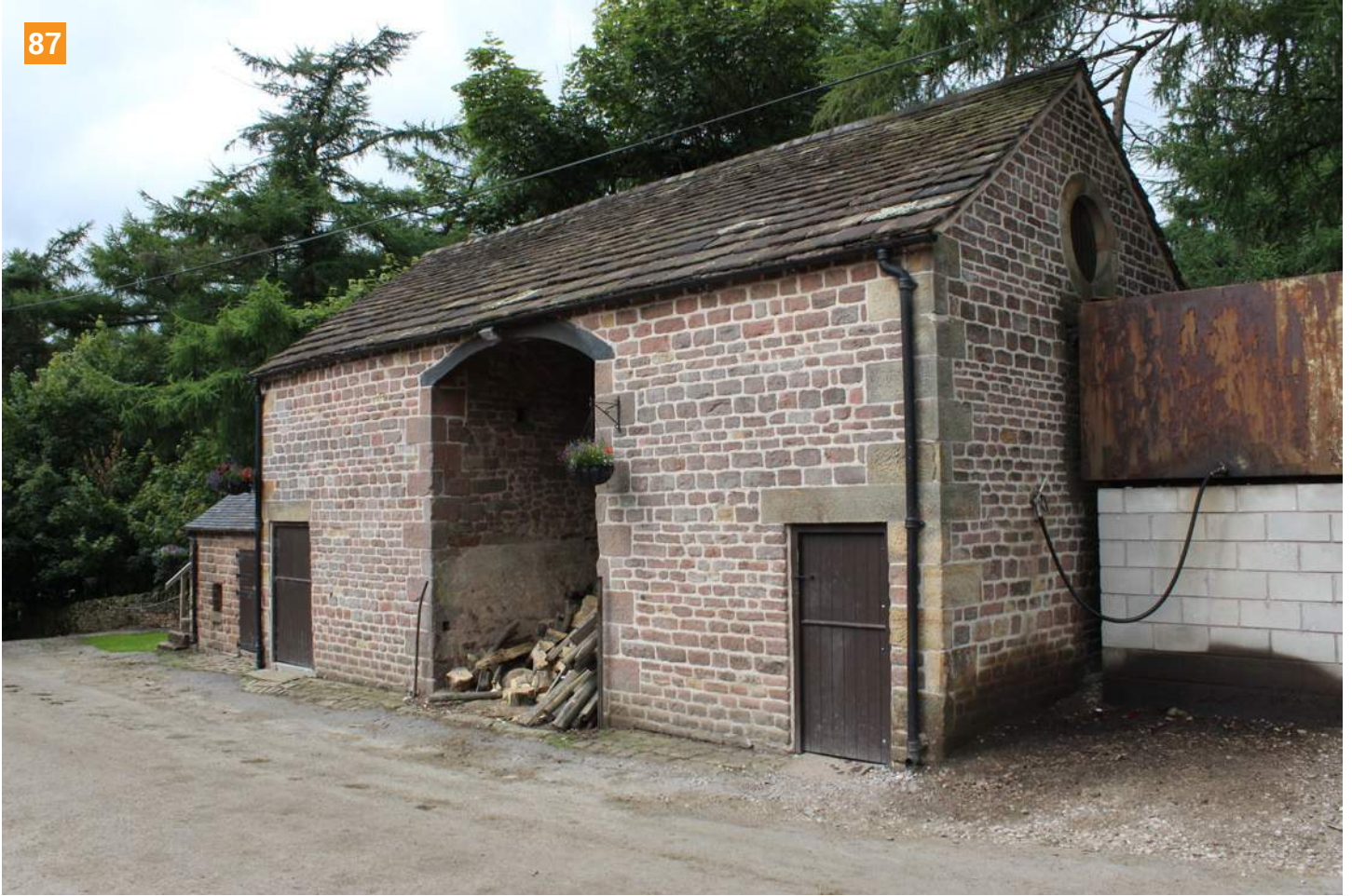
▲ 87. Stables set either side of a central open bay which probably housed a trap or carriage (South West Peak). Photo © Bob Edwards
