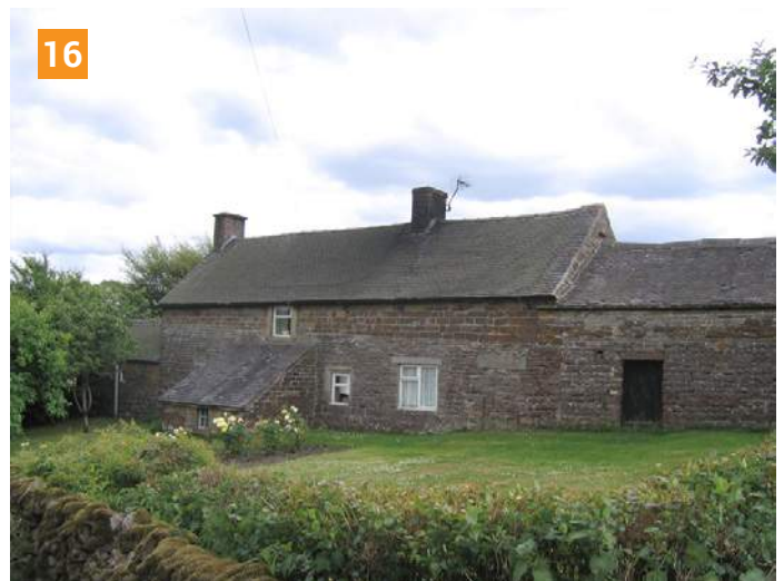
▲ 16. A Linear farmstead of in-line house and working buildings on the southern edge of the White Peak. Like many buildings, this shows the line of an earlier pre-19th-century single-storey range. Many buildings have earlier cores, marked by breaks in masonry and the lines of steeper roof pitches on the gable ends of buildings which have been heightened. Photo © Bob Edwards
