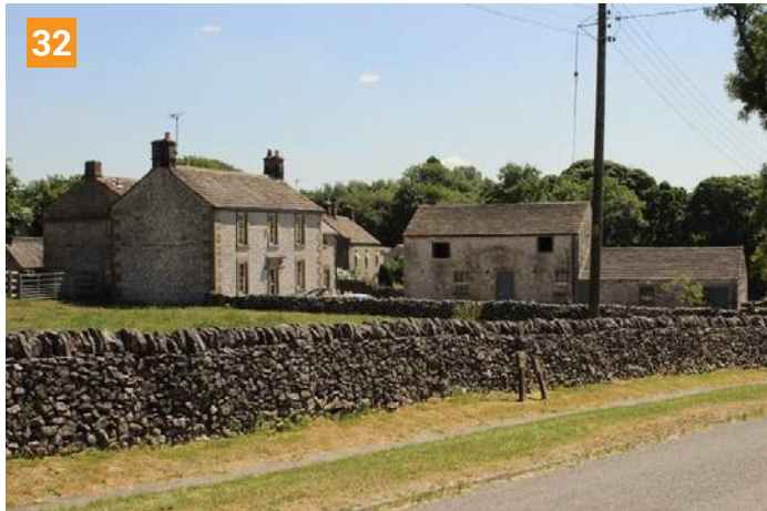
◀ 32. A Loose Courtyard with a building range to one side of an early 19th-century house, its fine symmetrical facade facing the road. The two-storey building was constructed as a combination barn, the threshing bay being later blocked and the building turned to serve solely as animal housing and hay storage. (Wormhill, White Peak) Photo © Jen Deadman
