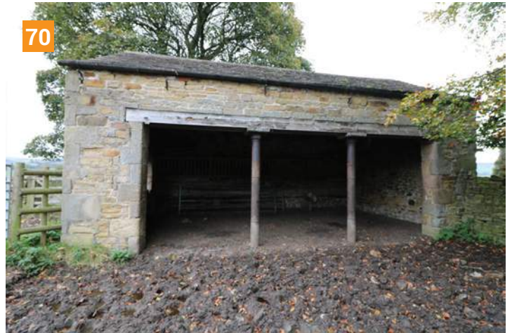
▲ 70. A shelter shed with cast iron columns, imported by rail into the Peak District from the mid-19th century and used on the Chatsworth estate as here. Photo © Adam Partington
