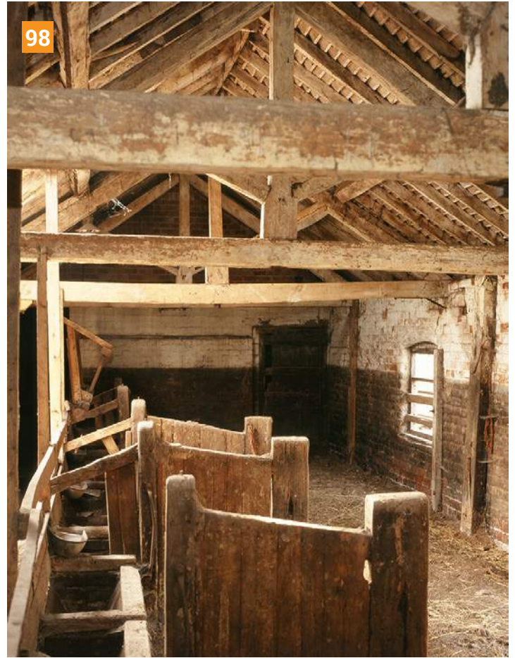
▲ 98. A more typical arrangement of cattle stalls and a manger with access to a feeding passage as found in single-storey cattle housing. Photo © Jen Deadman
