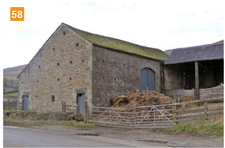
▲ 56. This early 19th-century threshing barn may have been built as a combination barn but it has been converted to serve as a cow house and hay store with the blocking up of the threshing bay – an alteration seen in several older barns reflecting the increasing importance of cattle over arable farming - and the later insertion of at least one of the first-floor openings (Wormhill, White Peak). Photo © Jen Deadman
