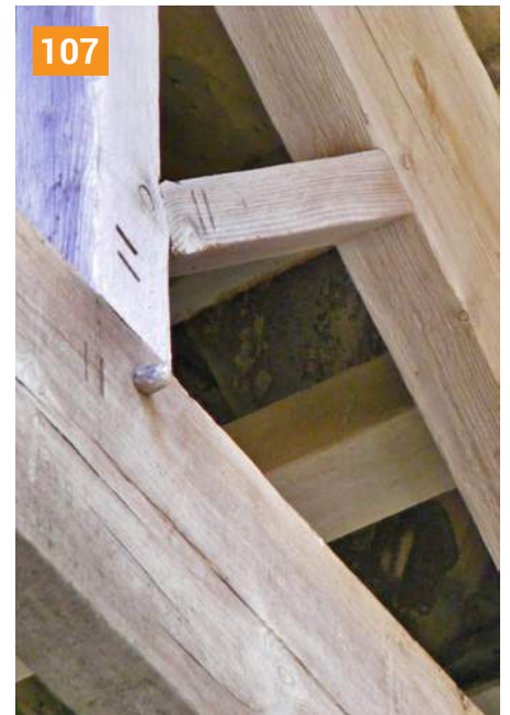
107. A carpentry mark for the assembly of pre-fabricated timber.
