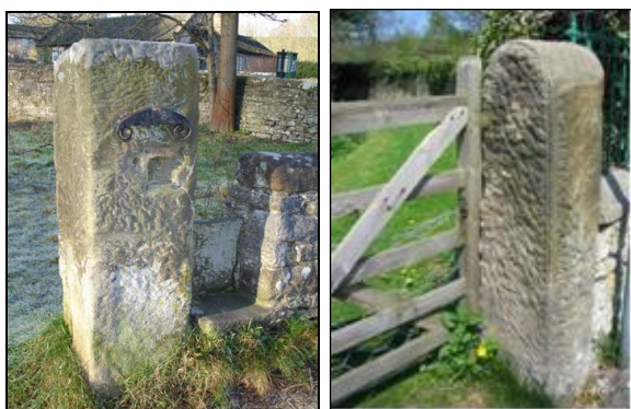
P.6.37. Left: Dressed stone gate-pier and stile
