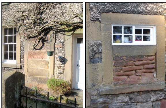
P.5.4. Left: Former entrance door, now blocked at Corner Cottage
