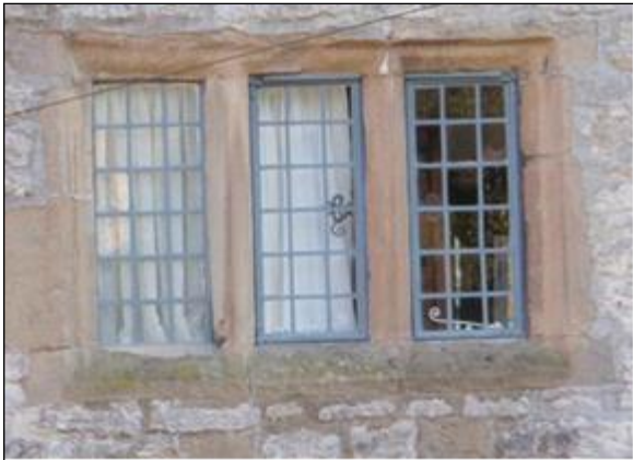
P.6.21. Double chamfered gritstone window surrounds and leaded lights, Monks Hall
