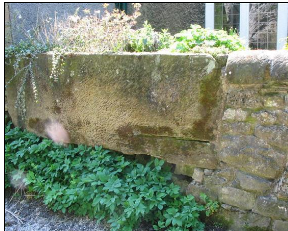
P.6.33. Trough forming part of the boundary wall, Rock Cottage
