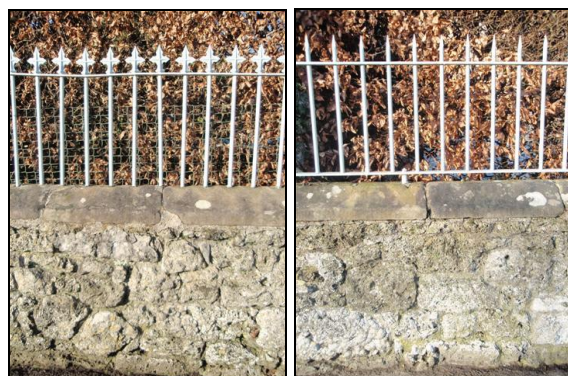
P.6.40. Left: Historic railings.
