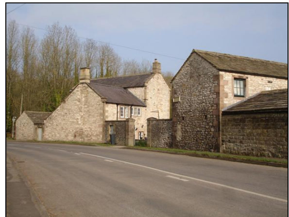
P.7.16. North-eastern edge of the main road
