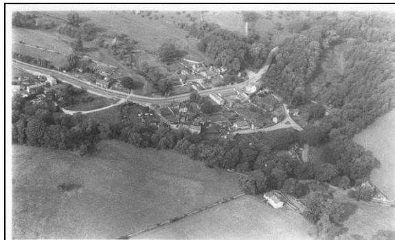
P.8.2 An Aerial View of Alport circa mid 20th century shows the extent of surrounding woodland © PDNPA
