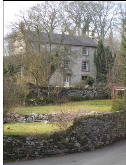
P.5.24. The front façade to Haddonfields partially screened by trees
