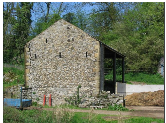
P.5.43. Open-sided barn, Rheinstor Cottage
