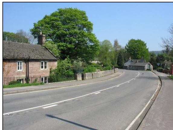
P.7.3. The main road from the west
