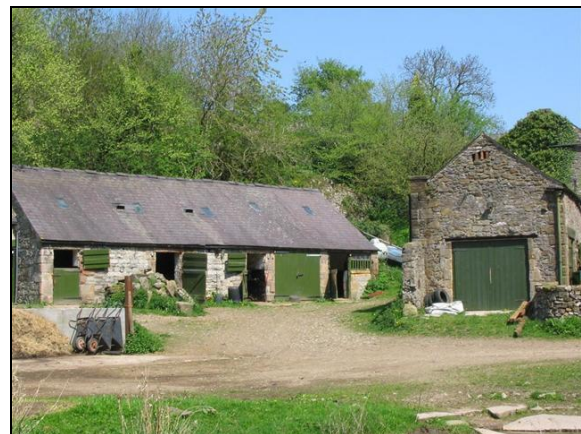
P.5.42. Stables & barn, Rheinstor Cottage
