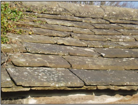
P.6.13. Stone slate roof covering
