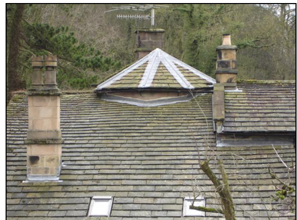
P.5.38. Complex roof forms, Rheinstor Cottage
