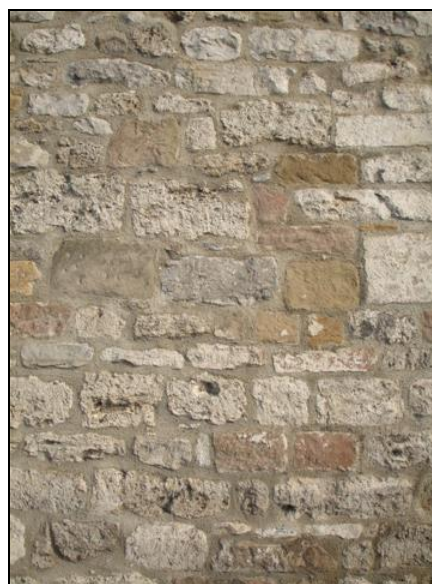
P.6.4. Limestone, tufa and gritstone form the rear wall to Haddonfields.
