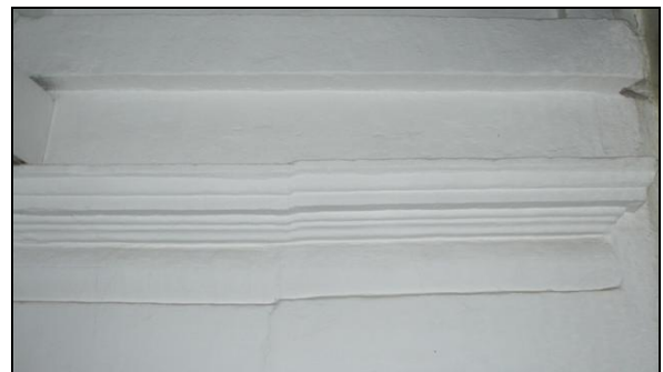
P.5.13. Classical label with stopped ends over internal doorway, Rheinstor Cottage
