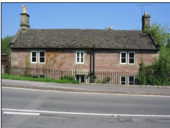
P.5.2. Front elevation of Lathkill Farm visually obscured by the higher road level
