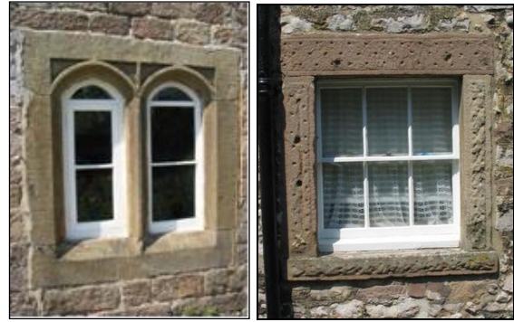
P.6.9. Left: Dressed stone window surround, Lathkill Farm
