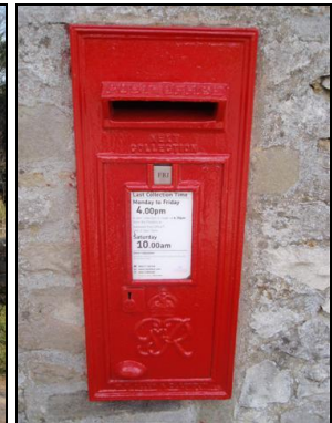
P.6.46. Right: Post-box in the back elevation of the Reading Room
