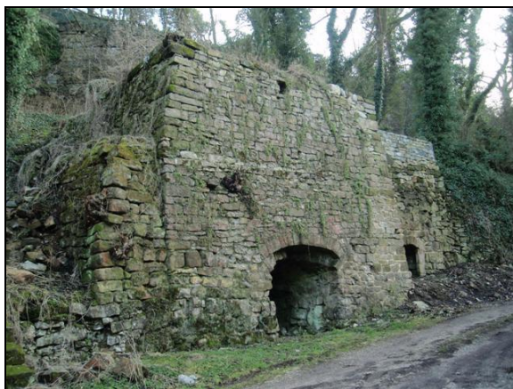
P.5.45. Limekilns east of the corn mill
