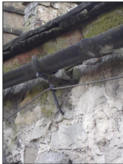
P.6.18. Drive-in gutter bracket with stay
