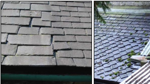
P.6.14. Left: Blue slate roof covering, diminishing and standard courses
