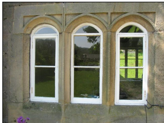
P.5.31. Ornate window surround in the east elevation of Lathkill Farm
