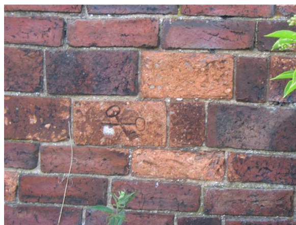
P.6.4. Imprint of keys within handmade brick outbuilding at Bell House, Uppertown.
