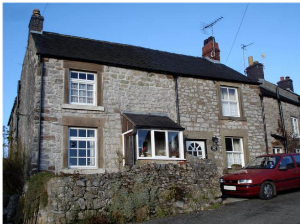
P.5.7. Part of the terrace along Bankside
