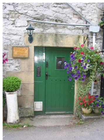
P.5.13. Principal Entrance to Dale House
