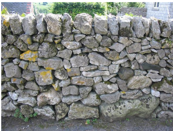
P.6.8. Limestone drystone wall
