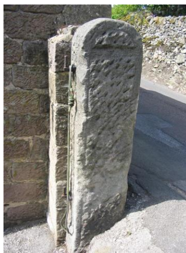
P.6.12. Broached tooling to gate-post at Hollies Farm
