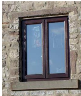
P.5.11. Re-used window lintel in the front of Lilac Cottage.
