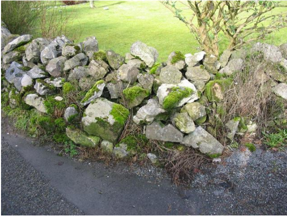
P.11.6. Drystone wall along Horsedale
