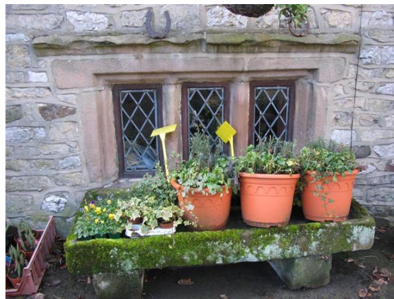
P.5.1. Double Chamfered Mullion Window at Hollies Farm
