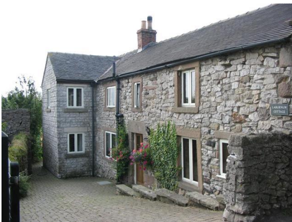
P.6.5. Davey block extension attached to Laburnum House
