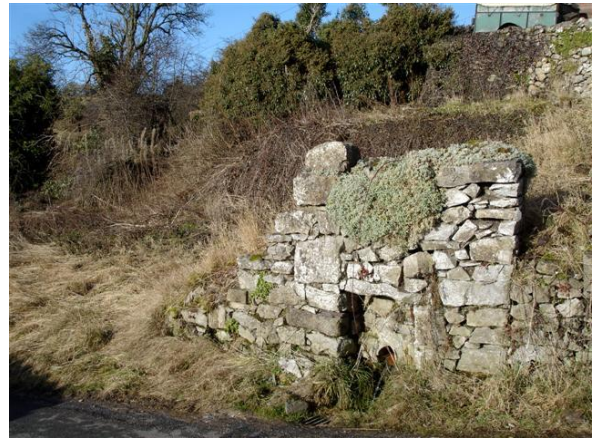
P.11.1. The well on Bankside
