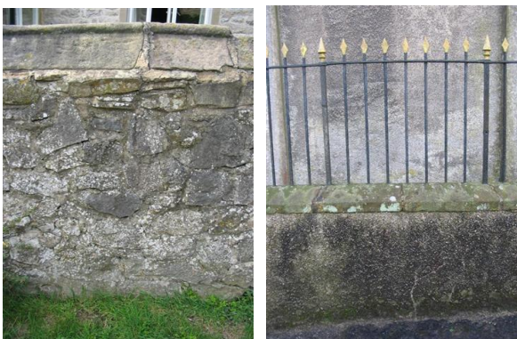
P.6.9. Left: Mortared limestone boundary wall with stone roll top copings
