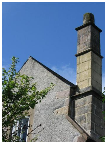
P.6.7. Three tiered chimneystack at Field Farm
