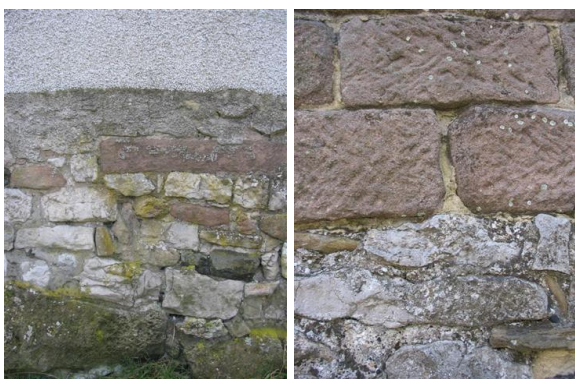
P.6.1. Left: Limestone and gritstone wall, built on bedrock and a wet dash finish above plinth level. P.6.2. Tooled gritstone above random limestone rubble
