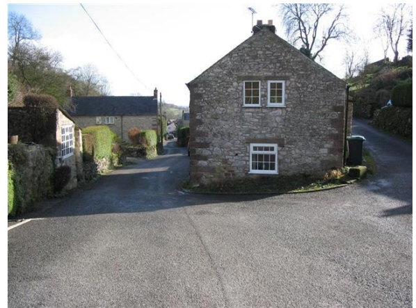
P.9.7. View down the Dale from the south-east corner of the Conservation Area
