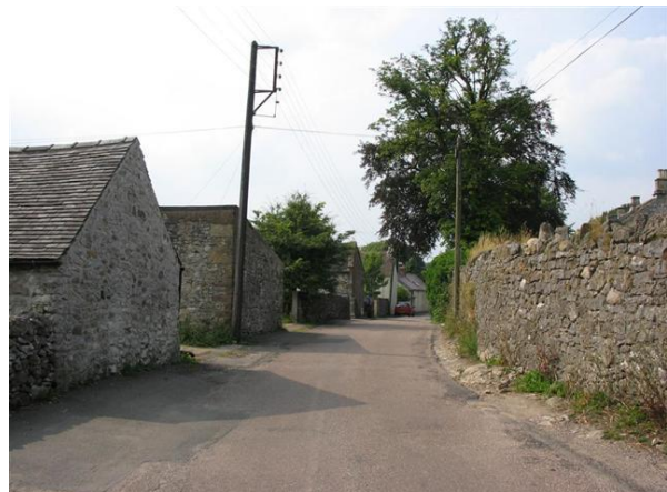
P.11.2. Overhead wires along Uppertown.
