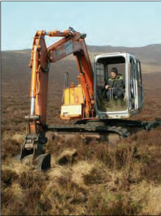
Contractor grip blocking on the Roaches
