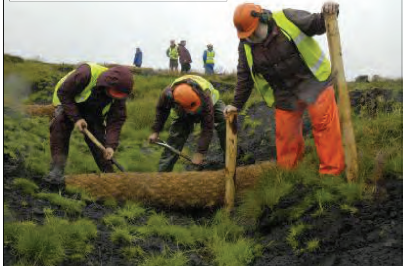
Coir rolls being installed on Bleaklow
