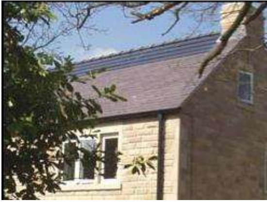
Figure 24. New build replacement dwelling, Curbar with simple arrangement of solar panels below the ridge
