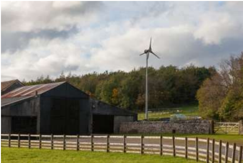
Figure 37. Example of turbine located close to buildings and facing into the prevailing wind
