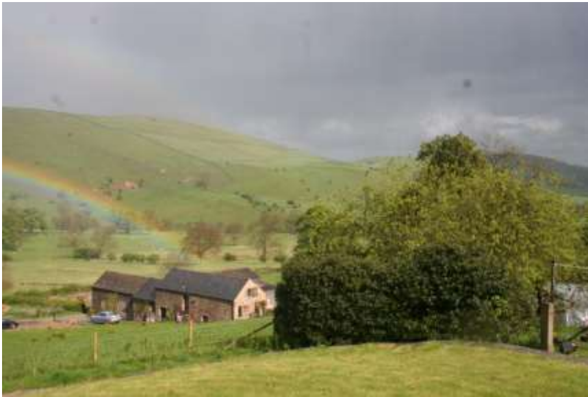
Figure 28. Dove Valley, minimal impact on the landscape through use of a ground source heat pump
