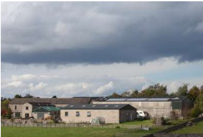
Figure 18. Solar Photovoltaics, Shallow Grange Farm
