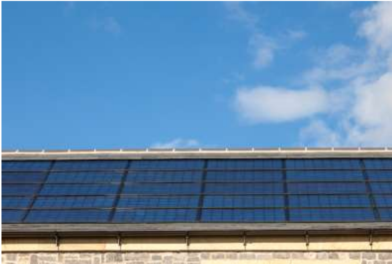
Figure 25. Flush fitted photovoltaic tiles
