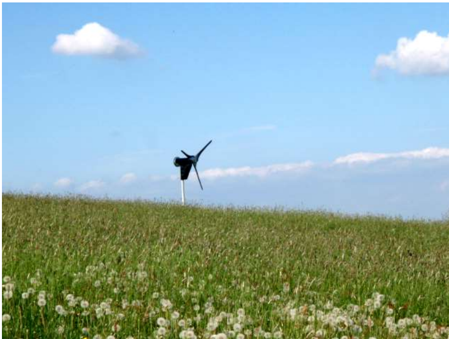
Figure 41. Example of a wind turbine breaking the ridgeline, demonstrating how skylining can impact negatively on the natural beauty of the area if the guidance in figure 35 isn't achieved
