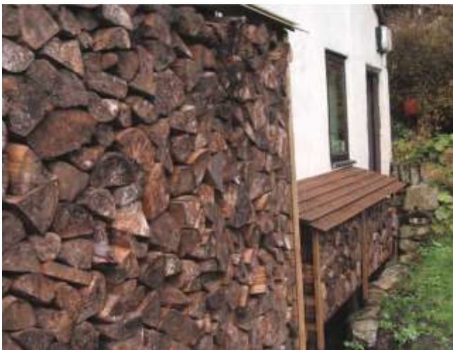
Figure 30. Wood fuel store for biomass stove
