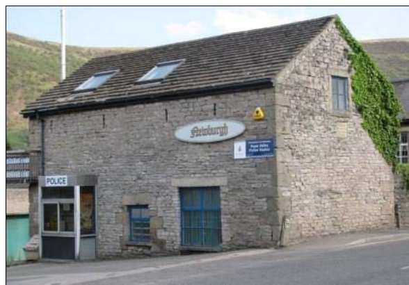
P3.3 The Police Station was formerly a barn
