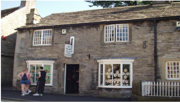
54 (above) This shop in Castleton relies only on hanging sign for signage
