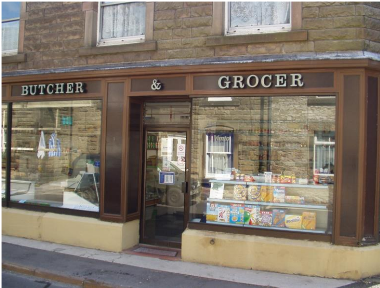
18 (left) Replacement shop front, Youlgreave (Church Street)
