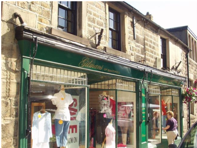
38 Projecting cornice incorporating traditional blind box
