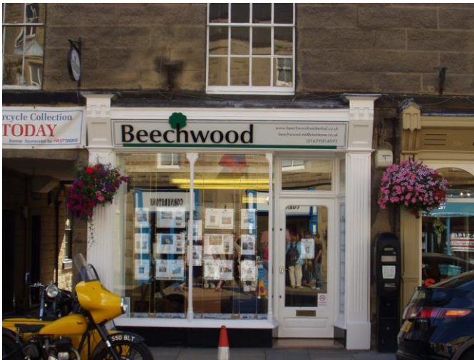
3 C19 shop front, Bakewell (Matlock Street)
