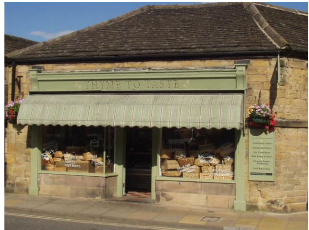
39 Original blind mechanism still in place
