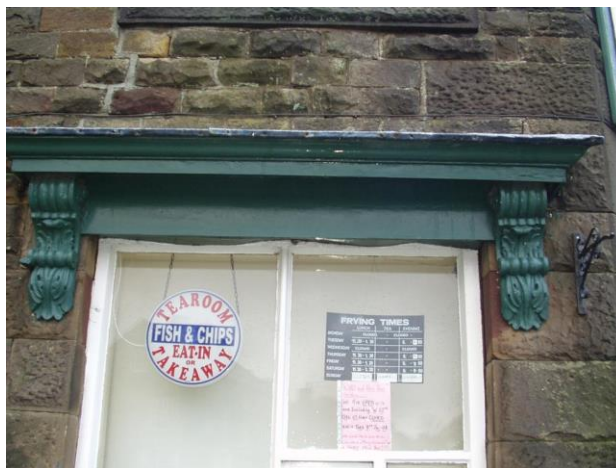
27 (left) Elaborate fluted console above pilasters 28 (above) Simple entablature in timber supported on timber consoles
