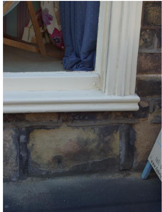
31 (above left) In this very simple Castleton shop front, the wall itself forms the stall riser
