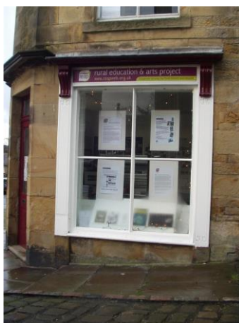
34 (left) Gritstone stall riser beneath simple subdivided window, Longnor
