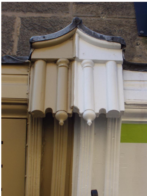
27 (left) Elaborate fluted console above pilasters 28 (above) Simple entablature in timber supported on timber consoles
