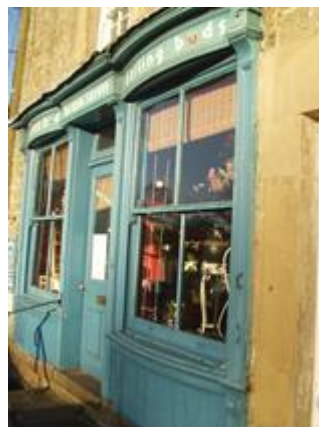
2 Shop front incorporating early details, Baslow (opposite Church on Main Rd)
