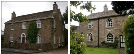
P5.13 Pott Hall Farm (left) and Church Cottages (right) both have Gothic windows
