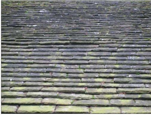
P6.7 Stone slate roof, St Christopher's Church
