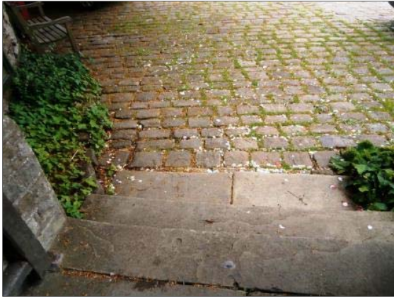
P6.21 Stone steps and setts in front of St Christopher's Church
