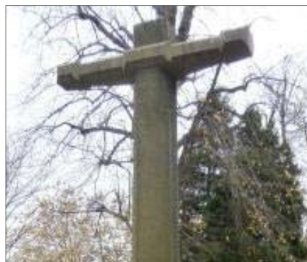
P5.6 The Cross transom is a later addition
