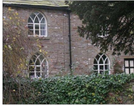
P8.17 Climbing plants help soften the appearance of walls
