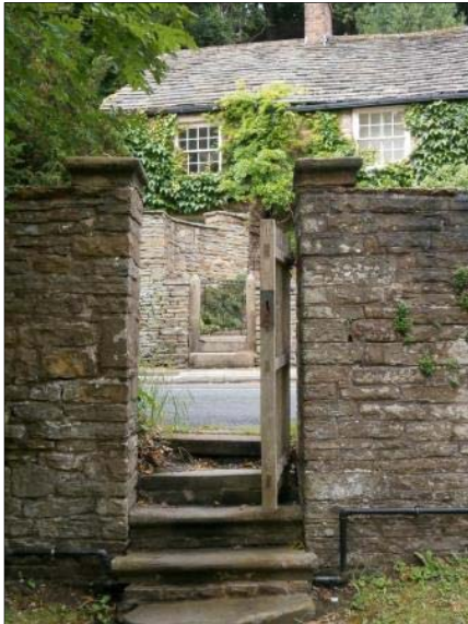
P6.1 Local stone has been extensively used for construction in Pott Shrigley
