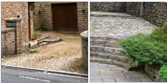
P6.22 (left) Setts at the entrance to Walkers Green and P6.23 (right) setts and flags in front of Pott Hall Farm
