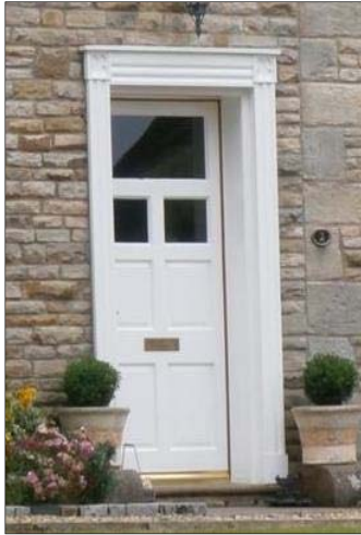
P5.11 Eighteenth century doorway at Pott Hall
