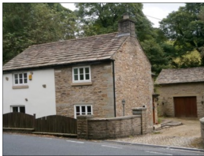
P5.8 Woodbine Cottage (above) and Walkers Green Cottage (below)
