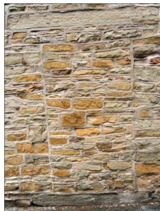
P5.7 Evidence of a blocked doorway
