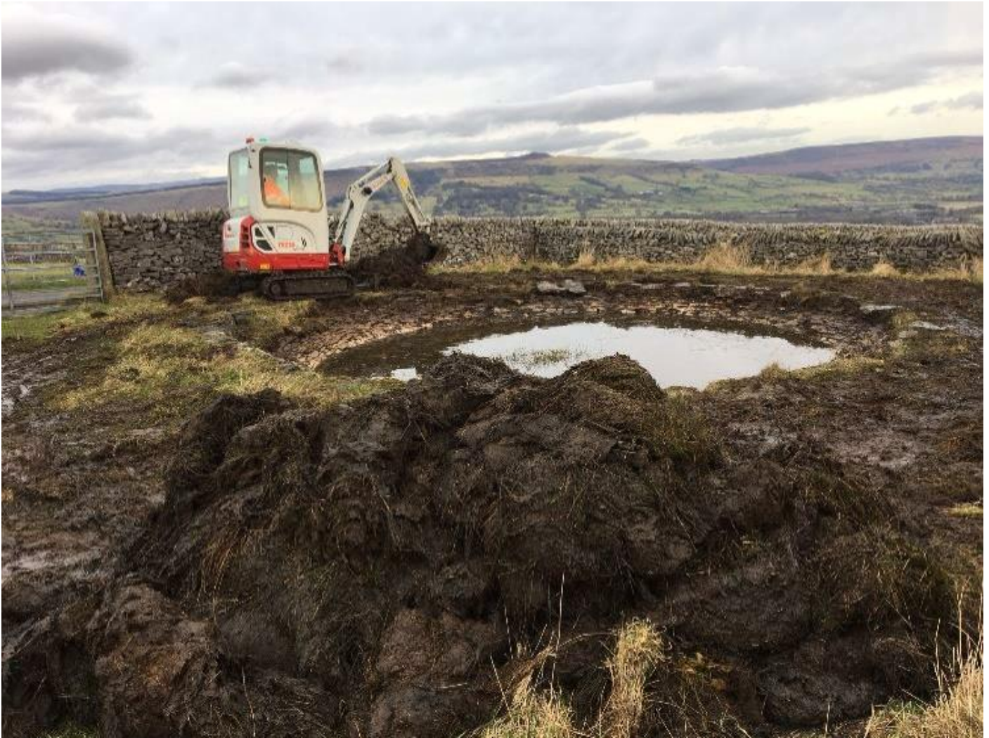
5 FiPL- Paradise Farm pond restoration - work in progress
