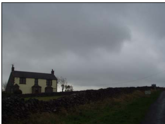
P50 Beacon House marks the start of the Village from the east
