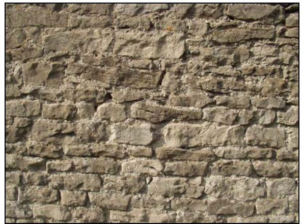
P36 Limestone rubble wall.
