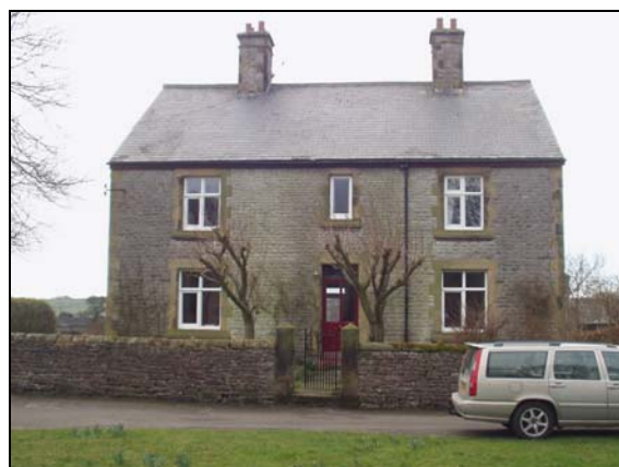
P11 Hall Farm, built on the site of the Manor House
