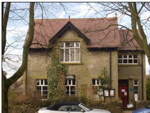
P55 Red clay tile, as used on the Village Hall, is not a traditional material
