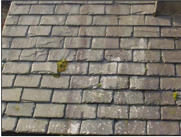
P33 Blue slate roof
