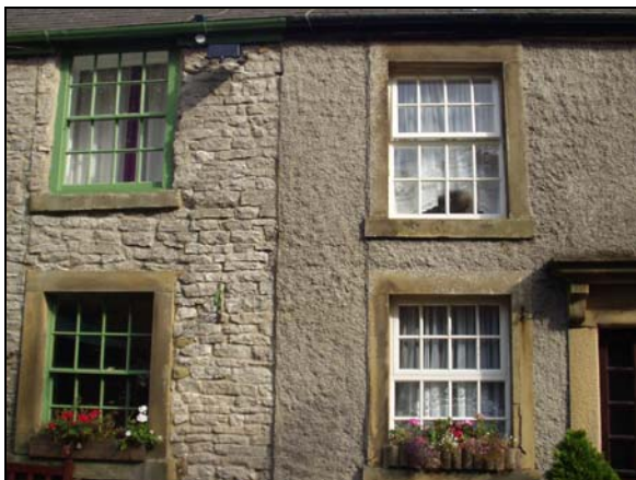
P37 Limestone wall and rendered wall with gritstone dressings.
