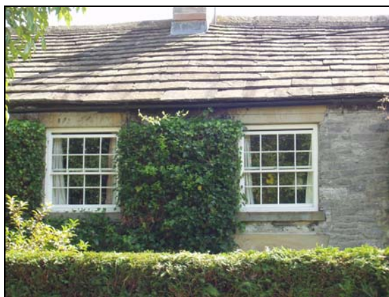
P29 Sash windows with stone heads and cills
