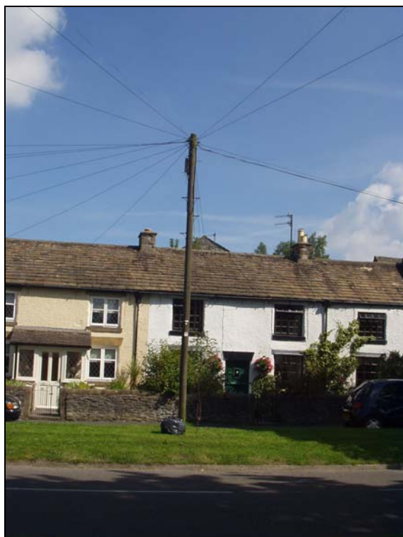
P54 Telephone wires on Main Street
