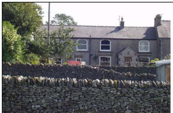
P22 West Villas with surviving sash windows
