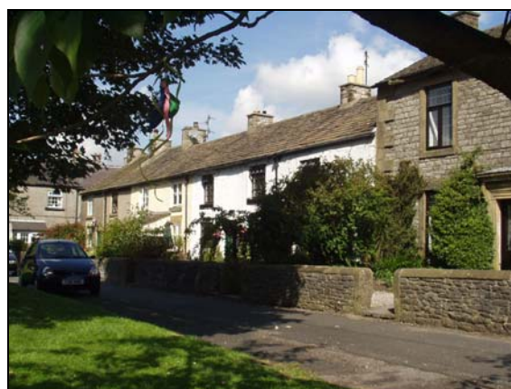
P25 Similar view showing some alterations.
