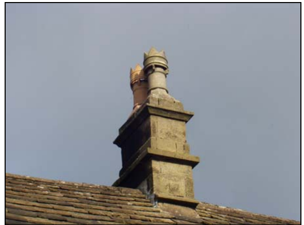
P38 Gritstone chimney on a stone slate roof.
