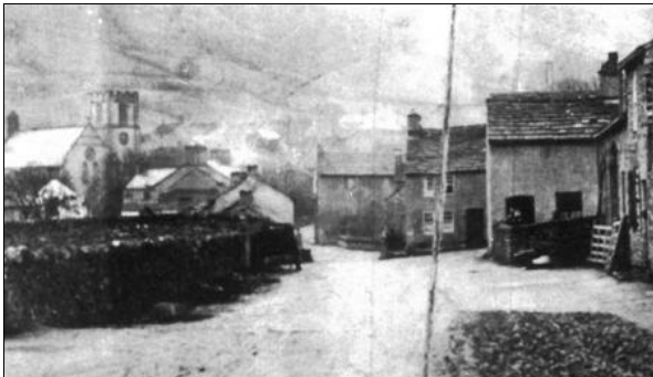
P4.3 Brook Buildings (centre) before conversion and addition of dormer windows
