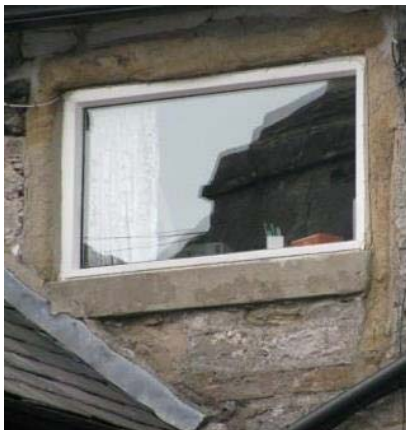
P5.7 Earlier window opening to 1 Towngate
