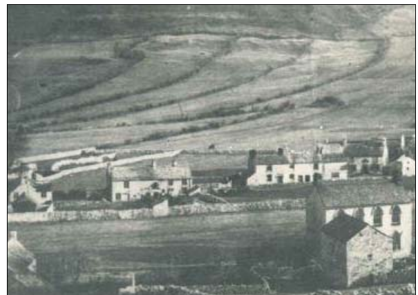
P4.7 Shoulder of Mutton (on the right-hand side, in the middle of the picture) before construction of the church
