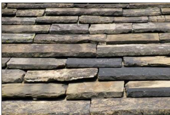
P6.7 Stone slate roof
