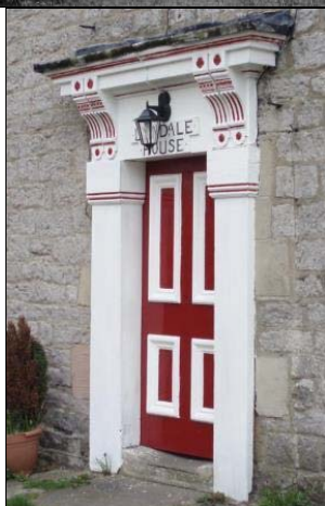
P5.39 Original door surround and windows at Lyndale House (top); doorcase today (bottom)
