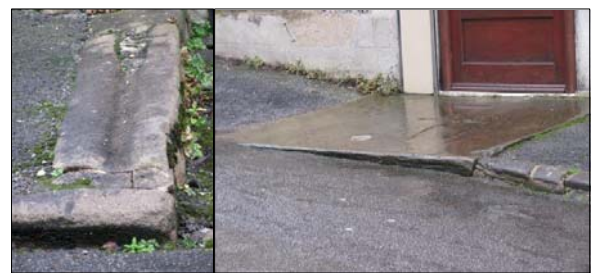
P6.17 Old Bull's Head: gritstone kerb with drainage channel, and gritstone threshold
