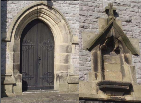
P5.26 Gothic detailing to Church of St. Barnabas
