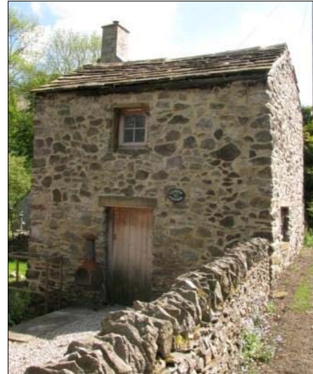
P4.4 Cannon Cottage, on Bessie Lane, was originally a hat shop
