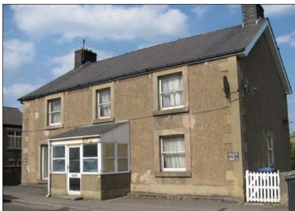
P5.23 Newburgh House today
