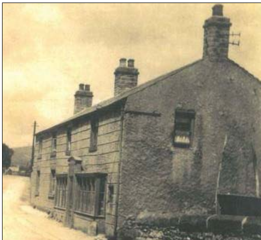
P5.12 Blocked earlier windows on the south-facing gable of Bridge House
