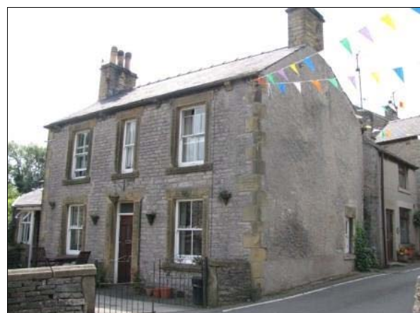
P5.30 A typical late C19th symmetrical frontage at Eccles View, Smalldale
