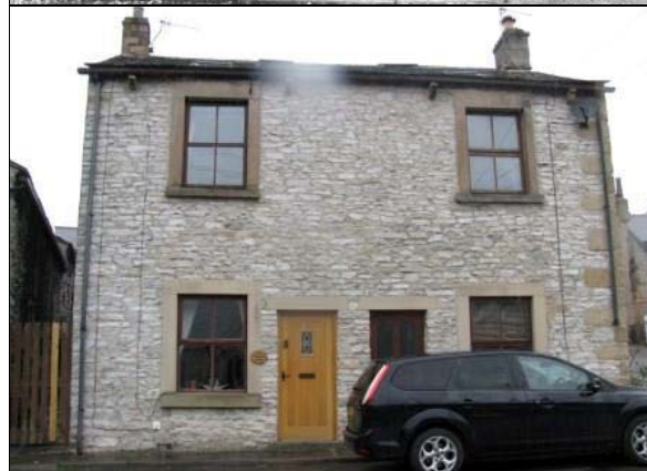
P5.46 Original shop front to 1 & 2 Towngate Cottages (top) and the cottages today (bottom)
