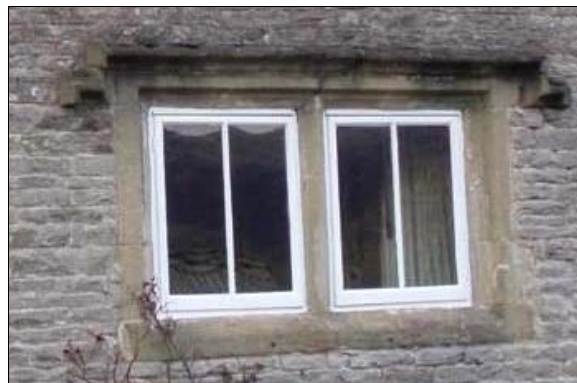
P5.4 C17th double-chamfered, mullioned window at Smalldale Hall
