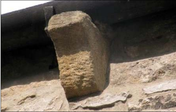
P6.3 Moulded gritstone corbel supporting gutter
