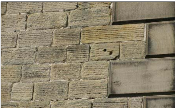
P6.4 Gritstone walls and quoins, Stanley House
