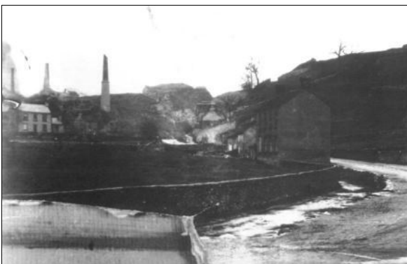
P4.1 Chimneys on The Hills, used as flues from the smelt works
