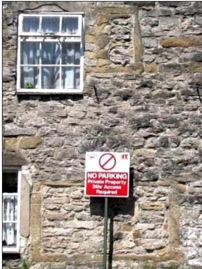
P5.12 Blocked earlier windows on the south-facing gable of Bridge House
