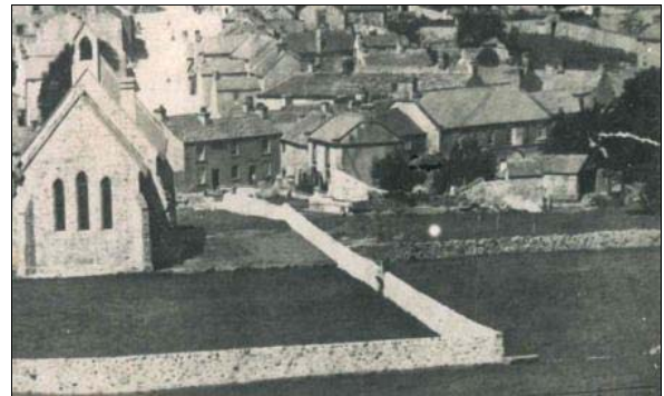
P5.17 Earlier, lower roofs to 1 & 7 Church Street
