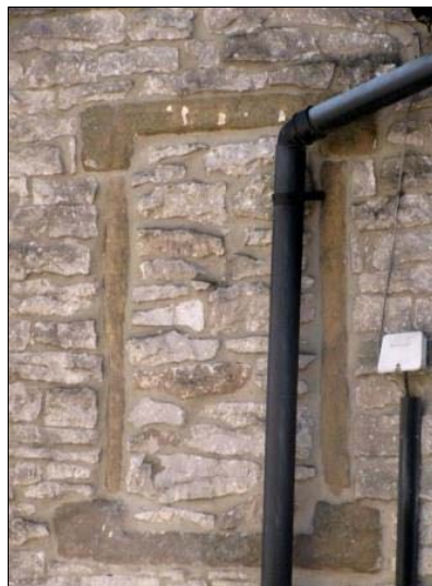
P5.21 Blocked C18th window to Hartle Cottage, Hugh Lane
