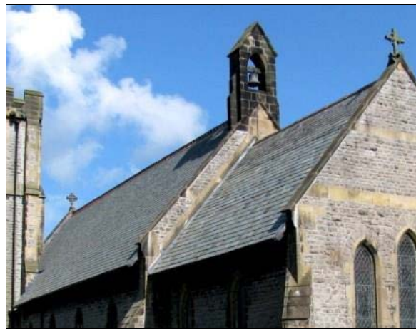
P6.8 Church of St. Barnabas roof - Westmorland slate
