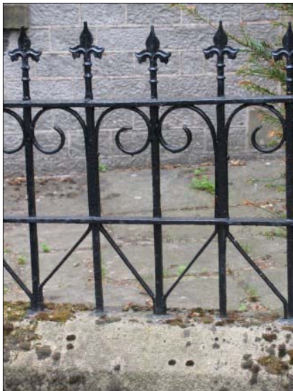
P6.14 Traditional railings at Dale View, The Hills
