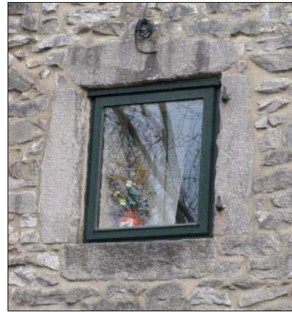
P6.5 Possible limestone window surround to mill building
