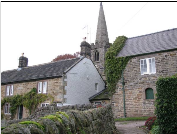
P5.12 The Old Bell House and The Bell Room are eighteenth century buildings.
