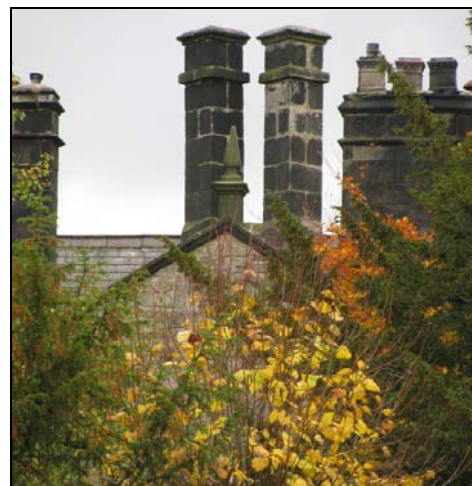
P6.4 Nineteenth Century Ashlar chimneys at Eastwood House
