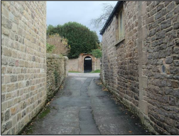
P6.6 A mixture of building and boundary walls on Besom Lane/Hall Lane.
