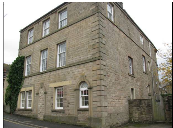
P5.14 Former Darvill's Mill Building dating from the nineteenth century, now converted into flats.
