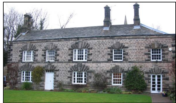
5.3 1830 Rock House with rusticated stonework to window surrounds.
