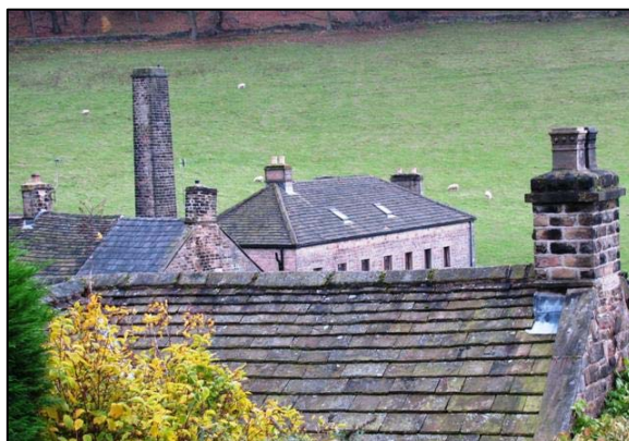
P7.5 Former Dale Mill building above rooftops
