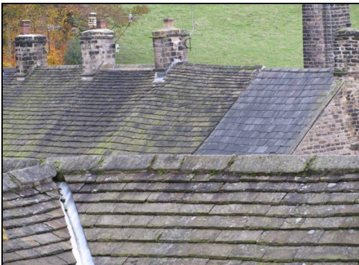
P6.2 Stone slate roofs and a blue slate roof
