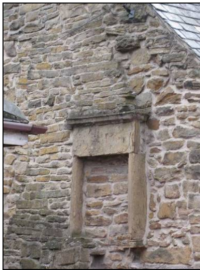
P5.6 A fireplace on the east gable of The Old Bakery, a former roofline can also be seen.
