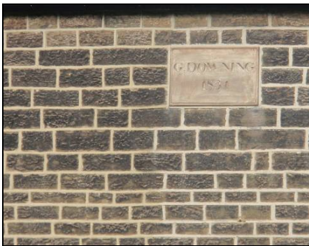
P6.1 Surface dressed coursed gritstone on Downing Row; note 1834 datestone
