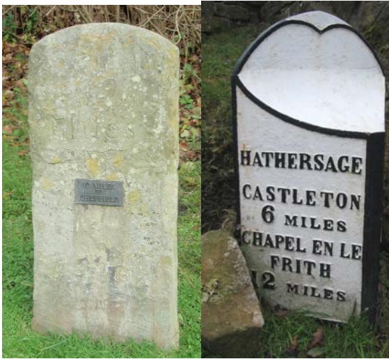
P6.10 Unlisted stone milepost and cast-iron listed milepost
