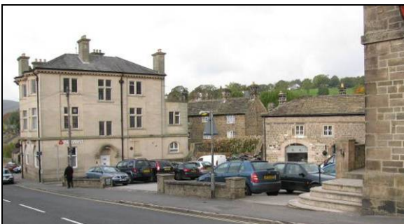
P5.2 The NatWest Bank stands out due to its scale, architectural style, and colour of stone.
