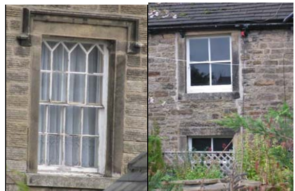
P5.10 Examples of early and late nineteenth century windows
