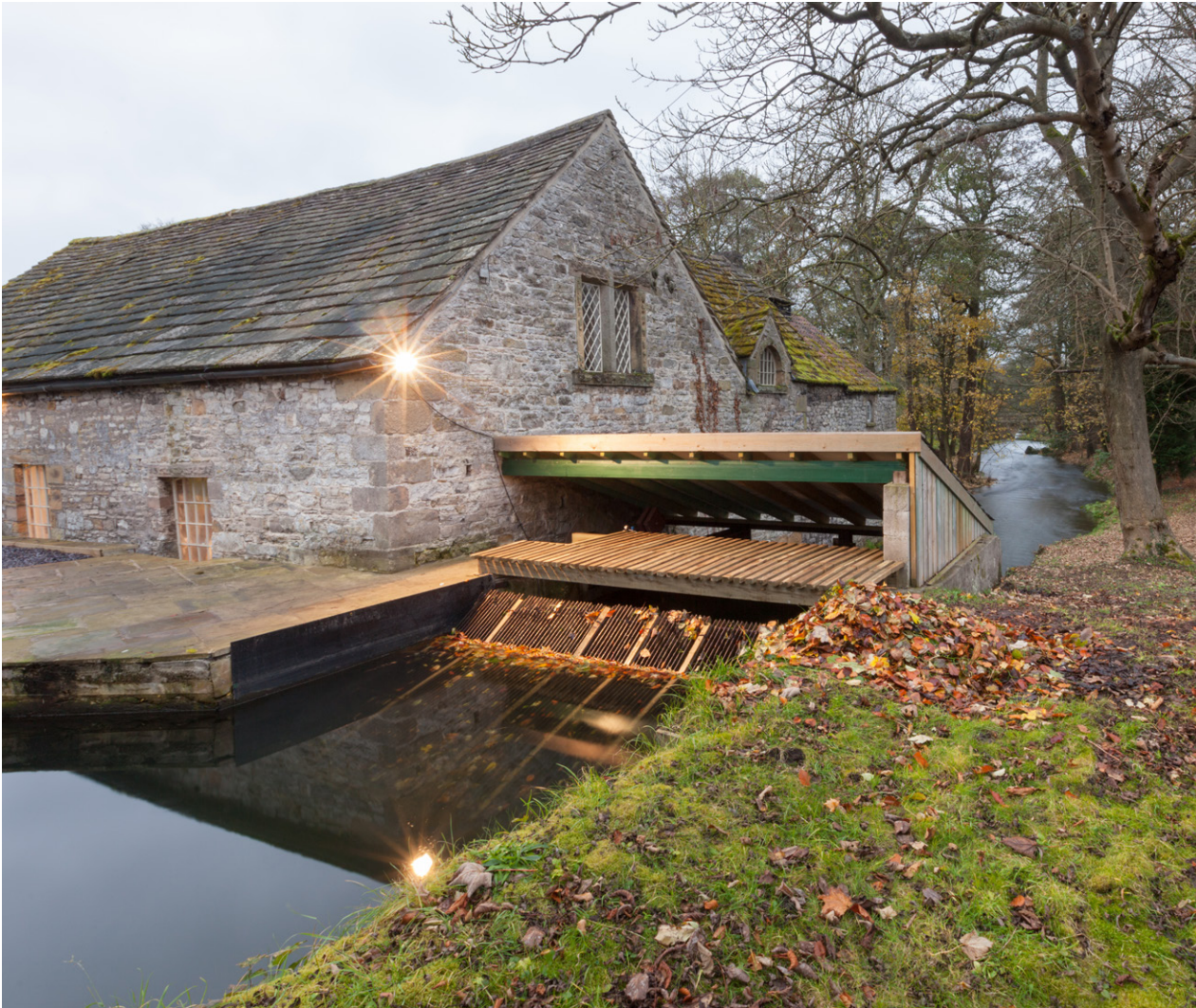
Figure 28. Flewitts Mill near Ashford in the Water
