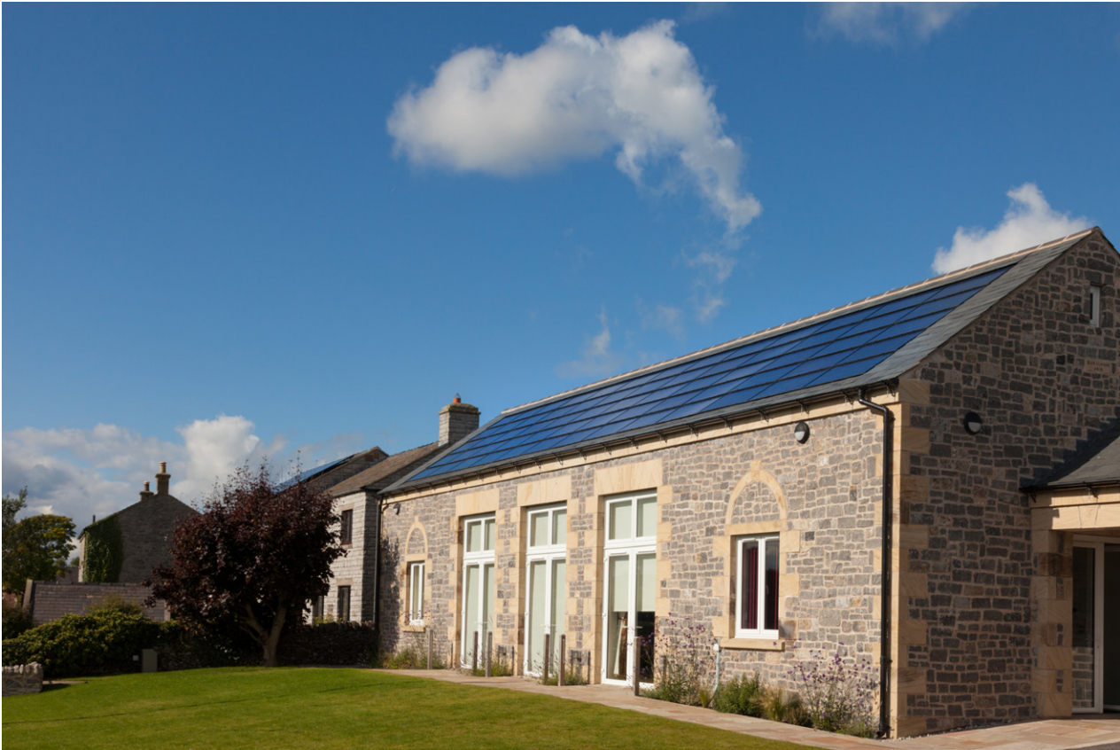
Figure 21. Over Haddon Village Hall
