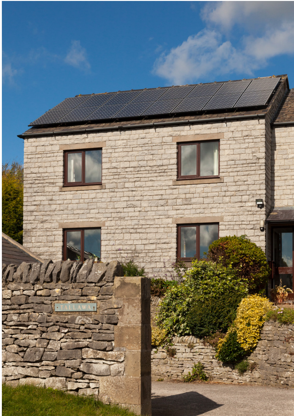
Figure 18. Retrofitted photovoltaics, Over Haddon
