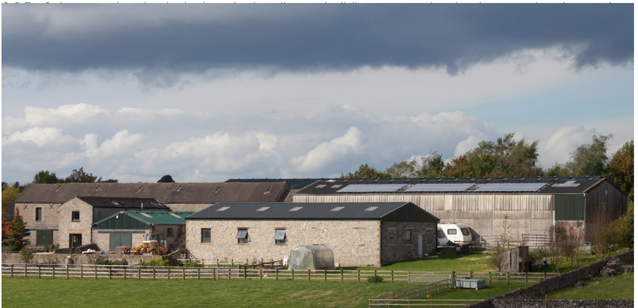
Figure 13. Solar Photovoltaics, Shallow Grange Farm
