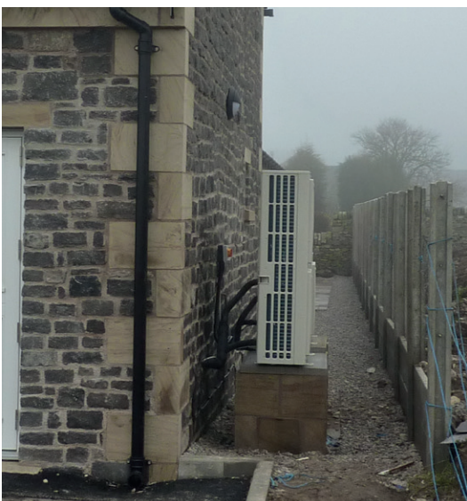
Figure 24. Air source heat pumps at Over Haddon Village Hall and on a new affordable home in Calver
