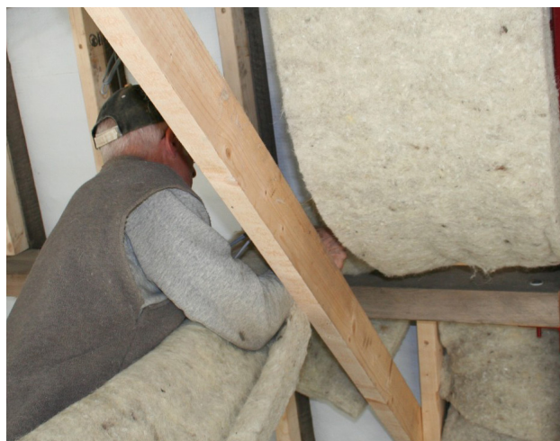
Figure 4. Sheep wool insulation
