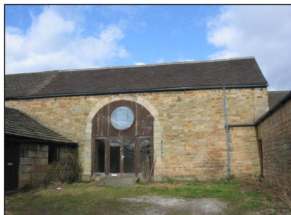
P.35 East end of Duke's Barn, School Lane
