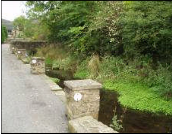
P.108 Piers lining Beeley Brook
