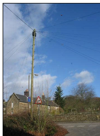
P.106 Overhead Wires, Church View
