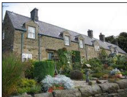
P.14 Chapel Terrace, off Chapel Hill
