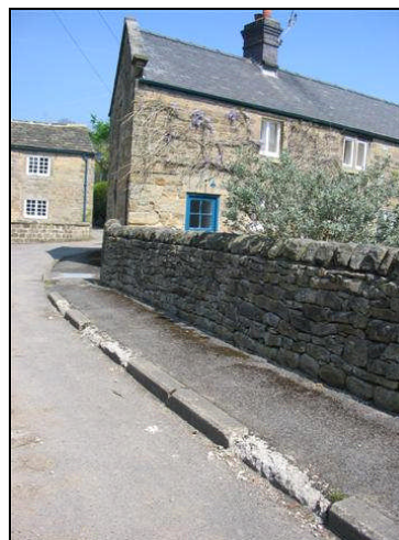
P.107 Concrete kerbs along Church View
