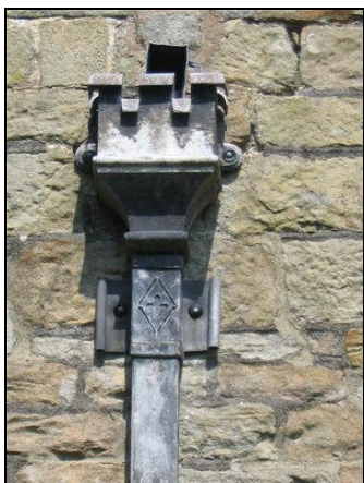
P.55 Lead Hopper, St. Anne's Church
