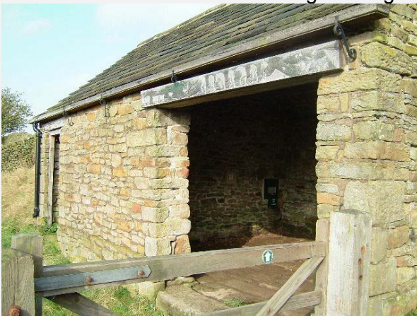
Photo: Structural use of timber in the UDV
