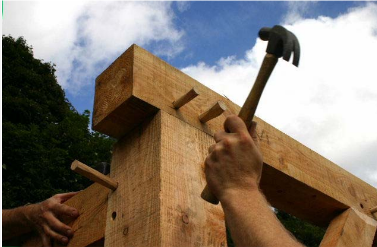
Photo: Timber frame construction (WWLtd)
