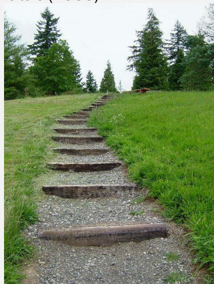
Photo: Timber steps (ECUS)
