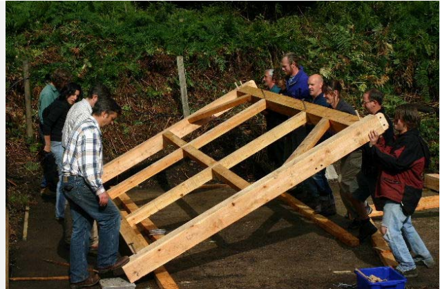
Photo: Timber roof frame (WWLtd)
