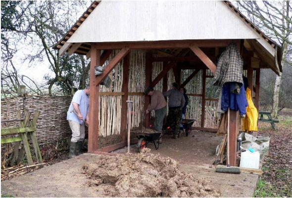
Photo: Timber and cob shelter (WWLtd)
