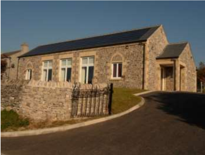
Figure 1. Over Haddon Village Hall
