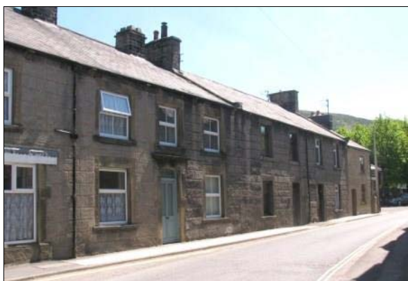
P7.7 The terrace of 1-7 Church Street leads the eye along the road in both directions
