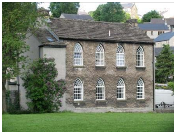
P7.26 Gothic windows of Brook House
