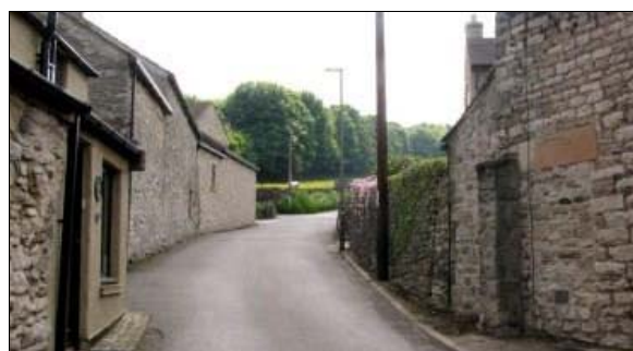
P7.9 The continuous walls of former barns at Hill Head
