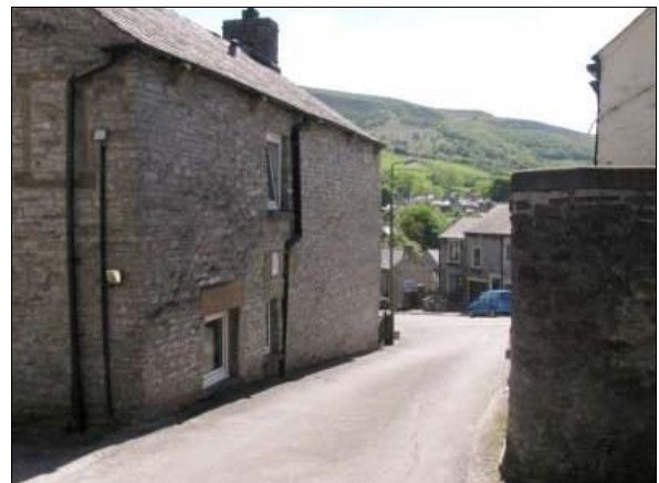
P7.16 The enclosed entrance into Towngate from Hugh Lane creates a sense of expectation
