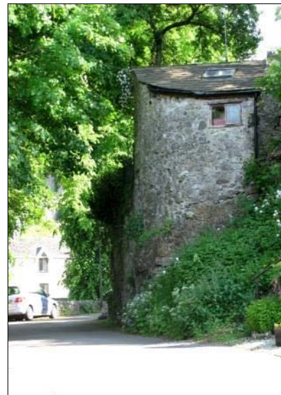
P7.31 Tower-like structure north of The Sett
