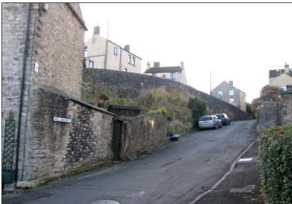
P7.38 Boundary walls dominate on Hollowgate
