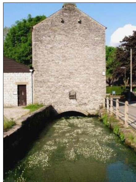
P7.21 Buildings span the Bradwell Brook
