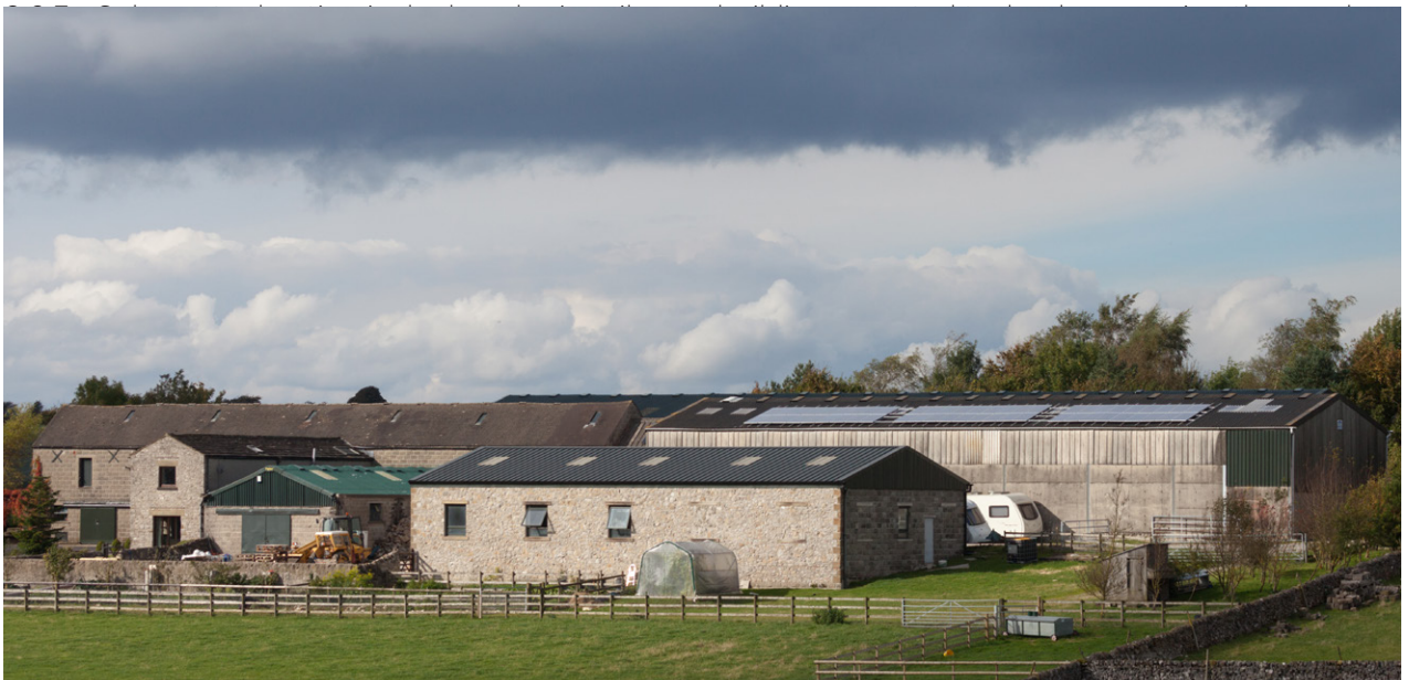
Figure 13. Solar Photovoltaics, Shallow Grange Farm
