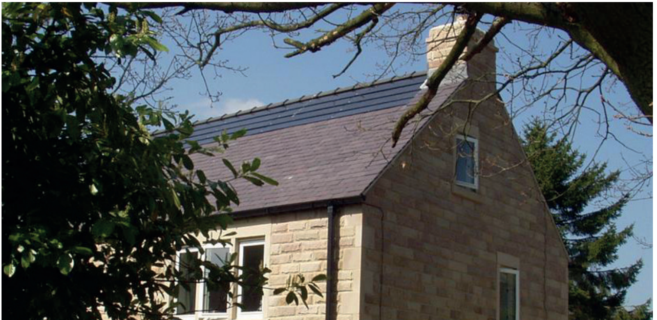
Figure 19. New build replacement dwelling, Curbar with simple arrangement of solar panels below the ridge
