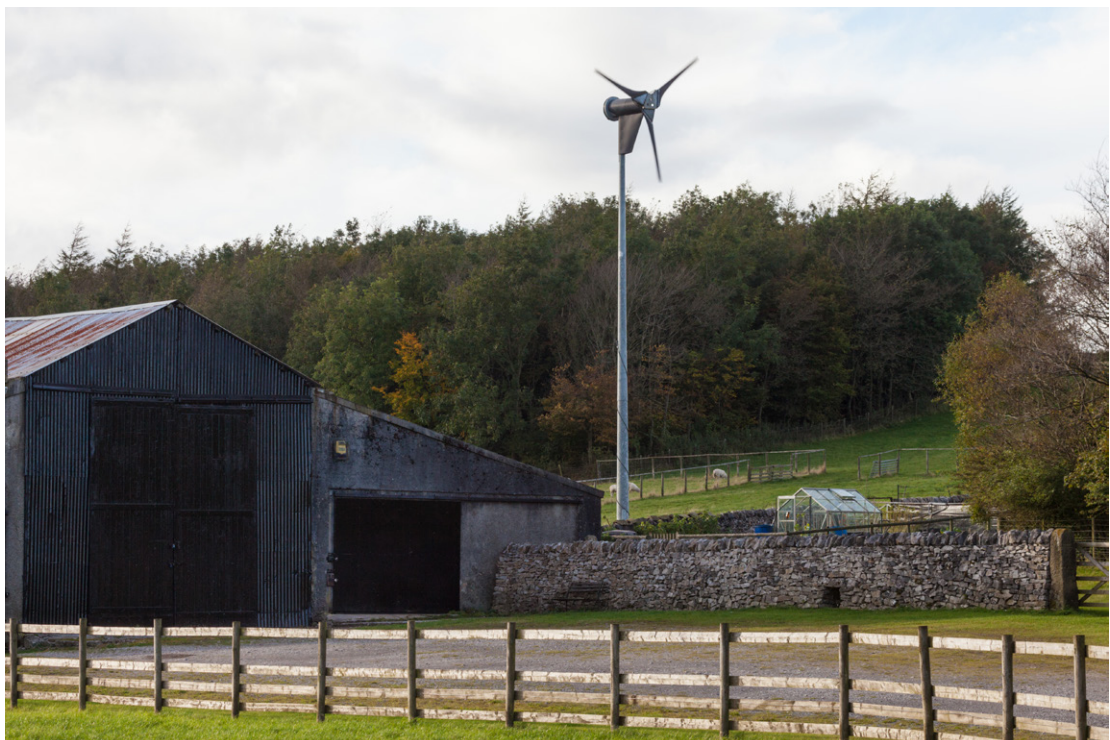
Figure 32. Example of turbine located close to buildings and facing into the prevailing wind
