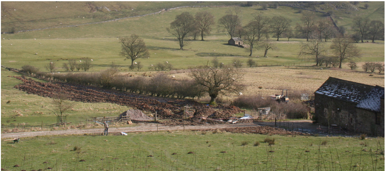
Figure 22. Ground source heat pump excavation
