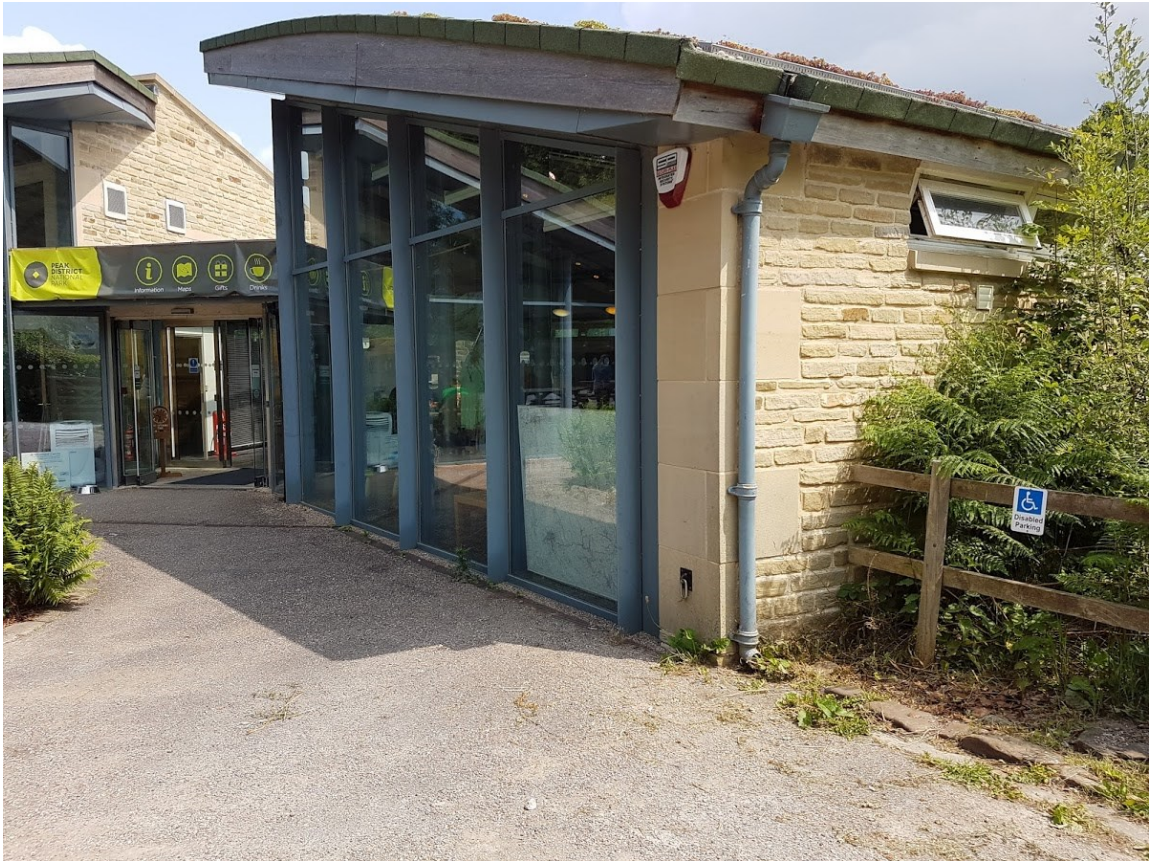
The path to the main entrance is gently sloping.
