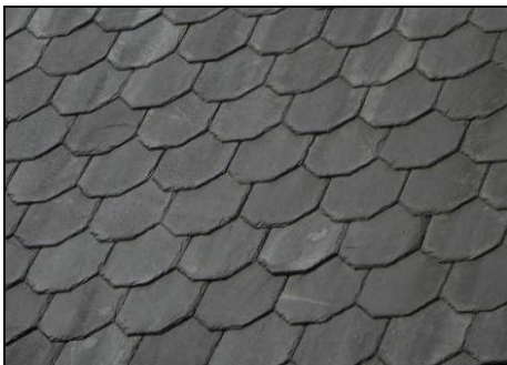
P6.2 Chamfered fishscale blue slates on Top Lodge
