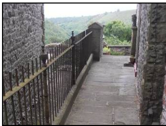
P6.13 Stone flags and railings, Middle Row
