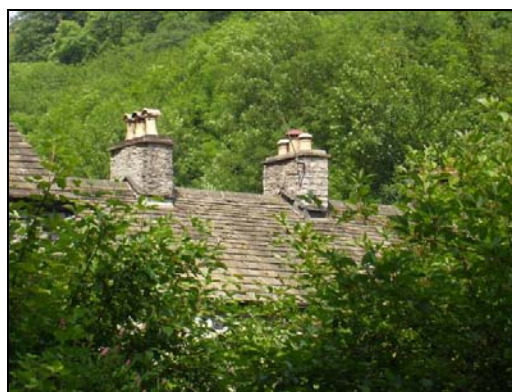
P8.7 The cottages are surrounded by trees
