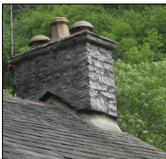
P6.7 Typical limestone chimney stack in Ravensdale
