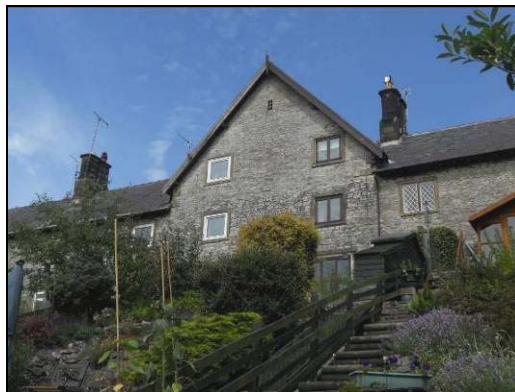
P5.4 Lower Wood Cottages
