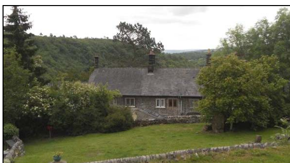
P7.18 The rear of Lower Wood Cottages from the Green, partially obscured from view.
