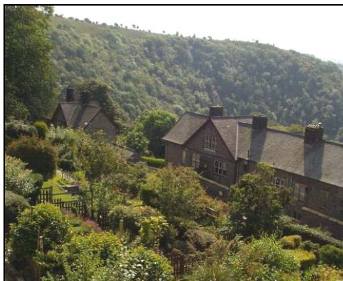
P8.3 The view from Top Row shows how trees impact on the village and it's wider setting
