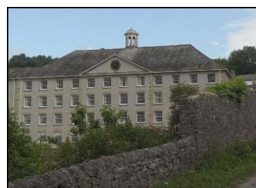
P3.1 The Mill constructed in 1816
