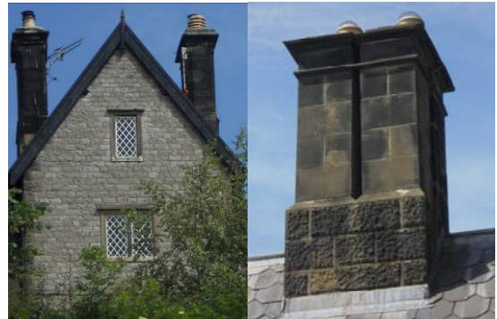
P6.6 Large chimney stacks in Cressbrook
