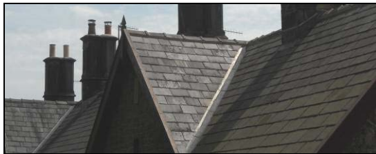
P6.3 Blue slate roofs on Middle Row
