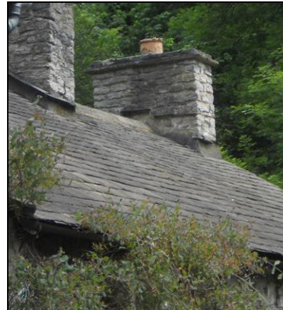
P6.5 Blue slate roofs found on 81-86 Ravensdale
