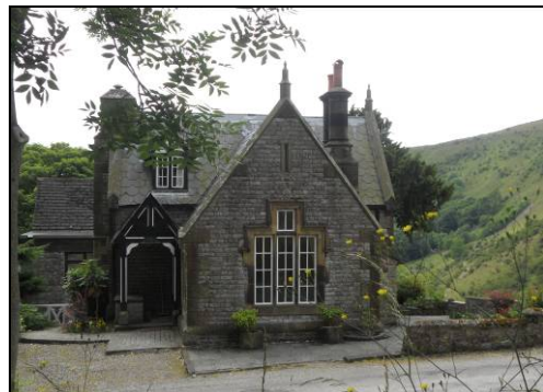
P3.5 Lower Lodge to Cressbrook Hall
