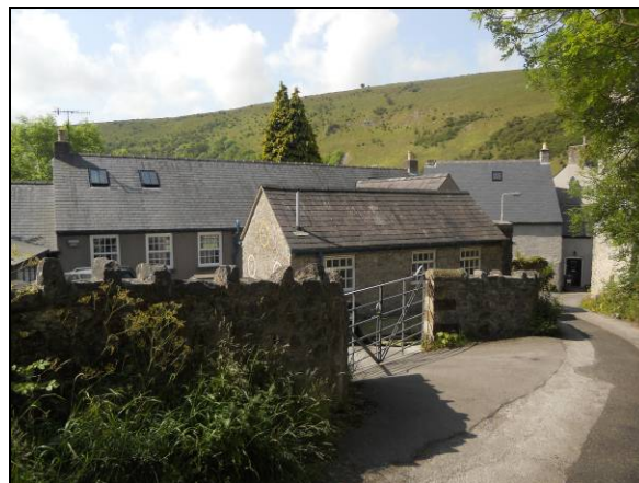
P7.6 The former school partially screened by walls
