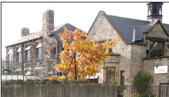
P4.2 The remains of the Atlas Works
