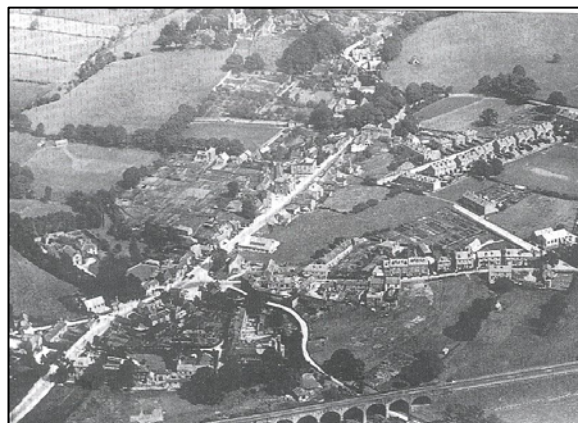
P3.5 Aerial photograph of Hathersage from the 1930s (reproduced with the kind permission of D. Upton)
