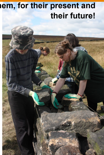
Youth Rangers building a drystone wall, an important heritage skill in the Peak District
