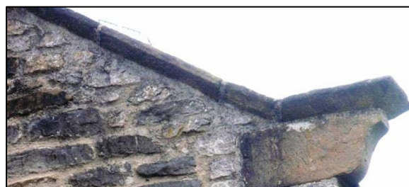
P32 Stone coped gable and moulded kneeler
