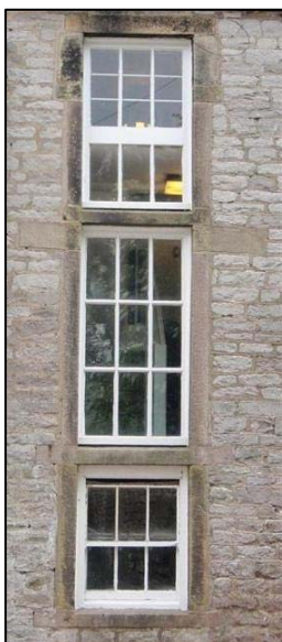
P34 Tall tier of lights to stairwell at Old Vicarage
