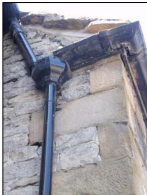
P43 Cast iron rainwater goods
