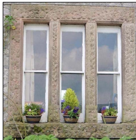
P36 Rusticated window surrounds to Hope View
