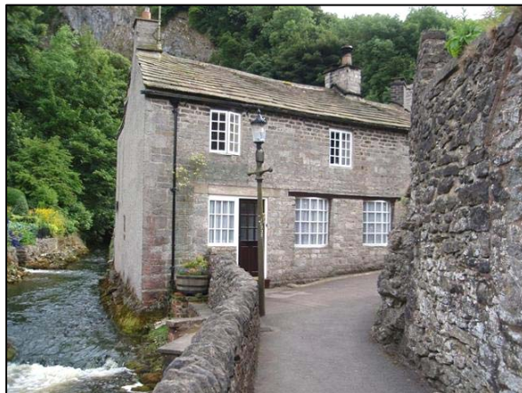
P79 Pinch-point by Hawthorne Cottage
