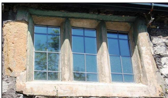
P27 Seventeenth / early eighteenth century window at Lodge Cottage
