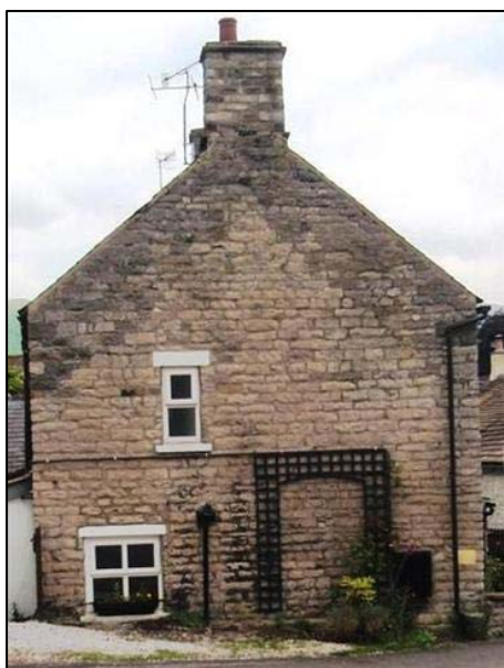
P30 Altered roofline at The Old Tea Room, Market Place
