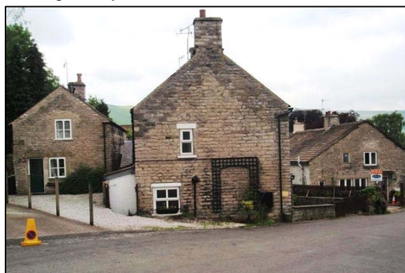
P59 Series of gable ends facing Bargate
