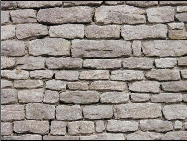
P47 Coursed rubble limestone walls
