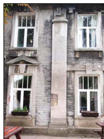
P28 Baroque features to Castleton Hall facade
