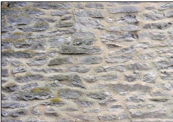
P48 Roughly coursed rubble limestone walls
