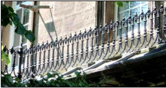
P45 Decorative iron balcony at Peveril House
