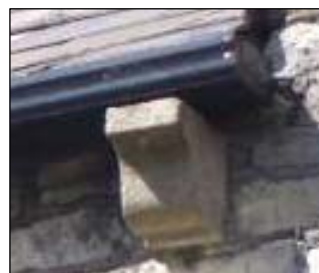
P33 Square section timber gutters supported on moulded stone corbels
