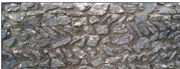
P24 Early Norman herringbone masonry at Peveril Castle
