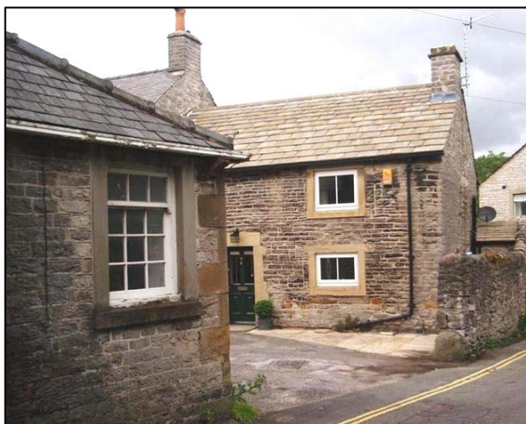
P18 Former agricultural building facing inwards towards former farmyard on Back Street
