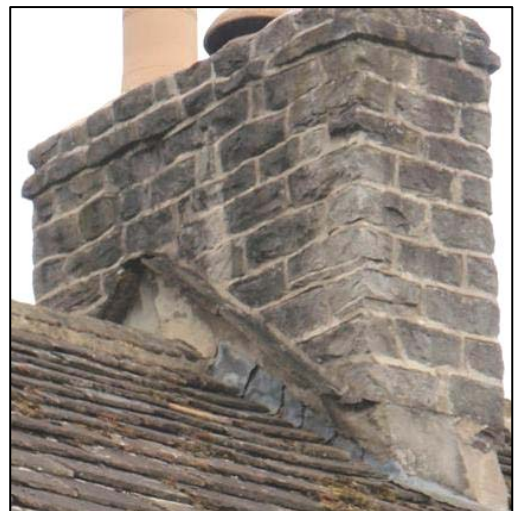
P52 Limestone chimney stack
