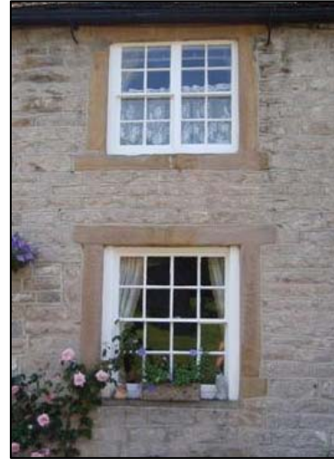
P40 Eighteenth century gritstone window surrounds
