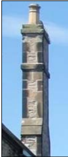
P42 Limestone chimney stack dressed with gritstone at The Castle Inn
