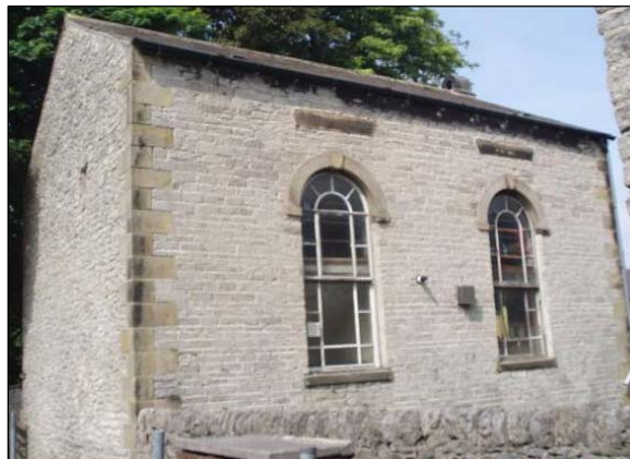
P14 Former Wesleyan Chapel on Back Street
