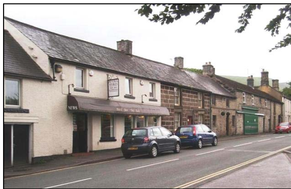
P21 Continuous terrace of adjoining properties on south side of How Lane
