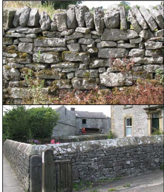
P6.6 Boundary walls
