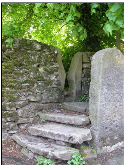
P6.9 Limestone steps at NE entrance to church
