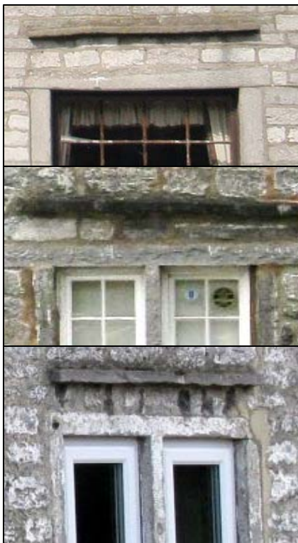
P5.4 From top to bottom: eighteenth century horizontal stone hood moulds at the Bull's Head, school and Shepley House
