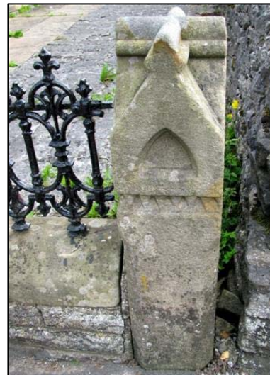
P5.11 Gate post + railings at Methodist Chapel
