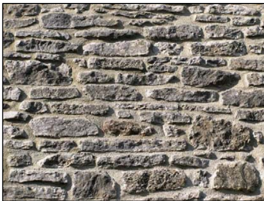
P6.1 Rubble limestone walling
