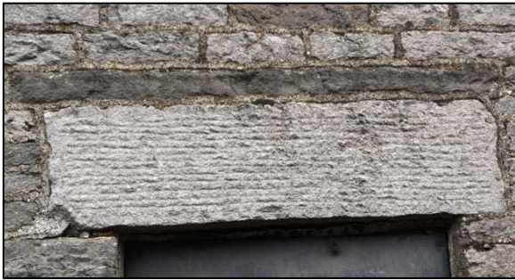
P5.9 Horizontal tooling to limestone lintel
