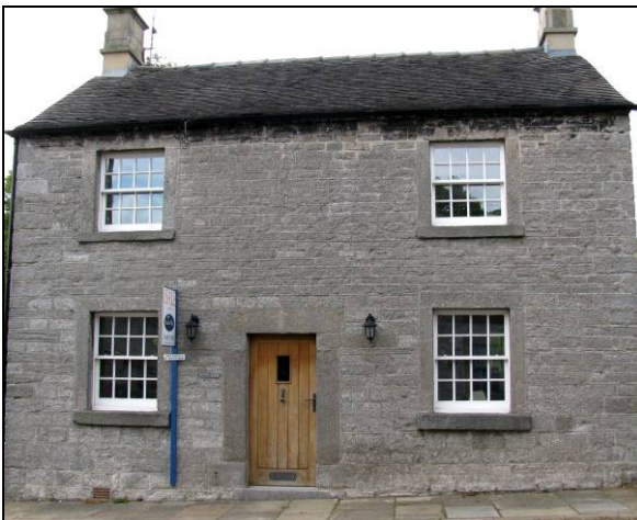
P5.10 Early-mid C19th windows at Bolton House
