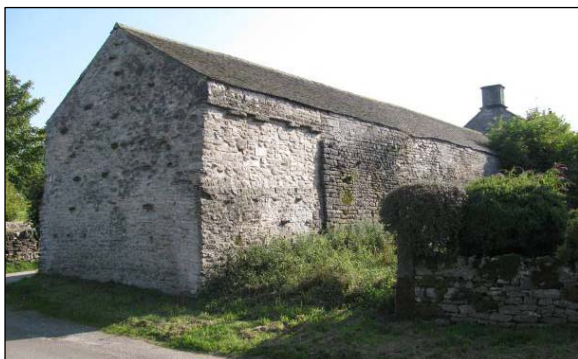
P7.20 Barn at Rake End Farm
