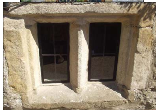
P5.3 Seventeenth century double-chamfered windows at Mount Pleasant (top); 1 Old Hall Cottages (bottom)
