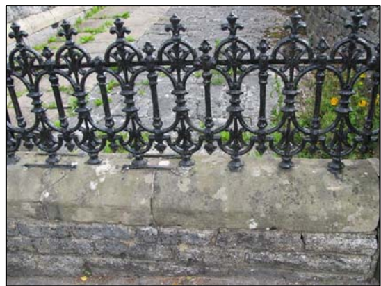
P6.7 Boundary wall+railings to Methodist Chapel
