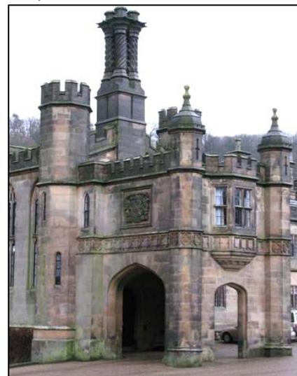
P5.4 Porte-Cochere at Ilam Hall
