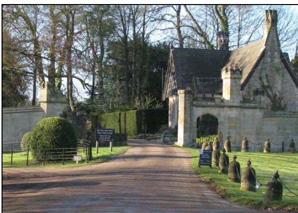
P3.12 Existing gateway to Ilam Park
