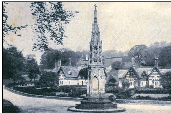
P5.12 Photograph showing the original tall, ornate chimneys to the cottages
