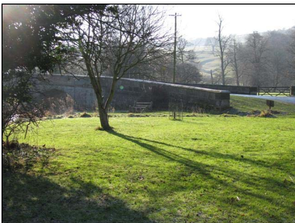
P7.7 Open views to south-east over the bridge
