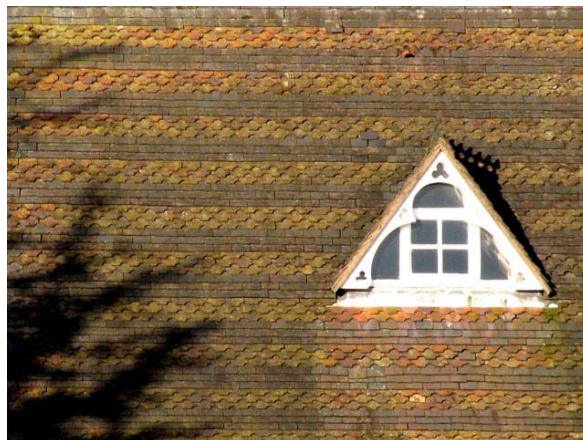
P5.11 Red and blue tiles to the school roof
