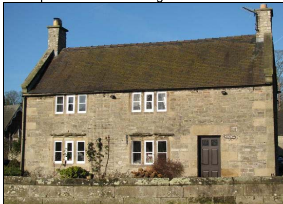
P5.2 Bridge View Cottage
