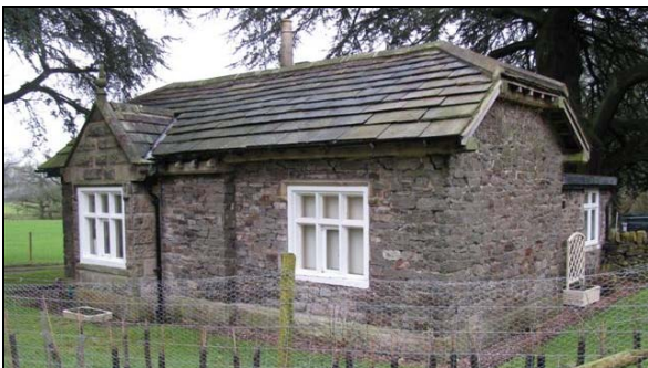
P5.6 Hipped stone slate roof to Church Lodge
