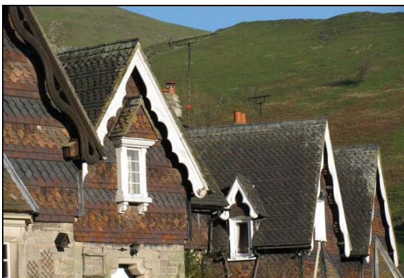
P5.9 Clay tile roofs and tile hangings to cottages
