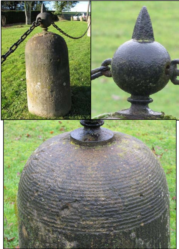
P6.4 Bollards beside the green outside Ilam Park entrance
