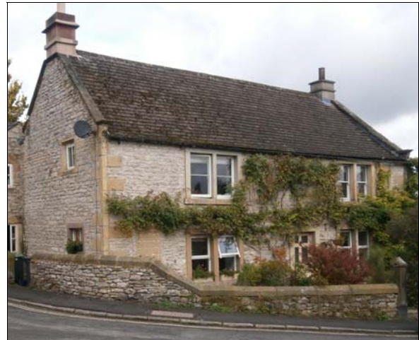
P4.11 Fellside, formerly the Bluebell Inn
