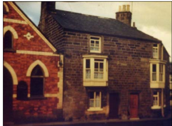
P4.14 The only available photograph showing the Primitive Methodist Chapel on Water Street, (on the left of the picture), before conversion
