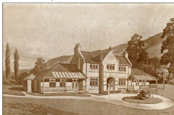
P3.30 The Bakewell Cottage Hospital
