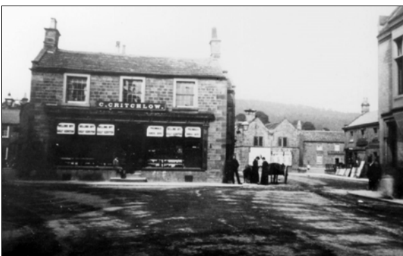
P4.10 Critchlow's shoe shop, demolished to make way for the new Post Office
