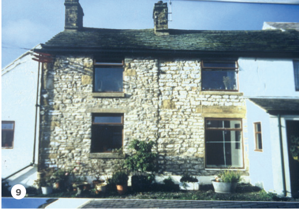
9: BEFORE: openings have been altered and original windows replaced in this cottage in Litton.
