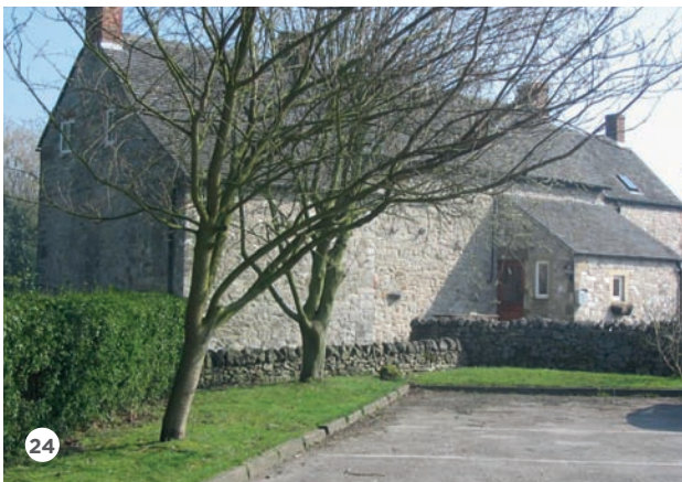
24: A modest, lean-to extension on the rear of a listed building in Parwich.
