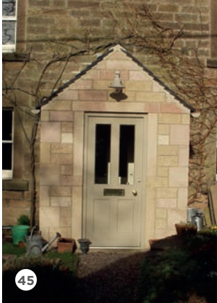
45: New stone porch with ridge roof
