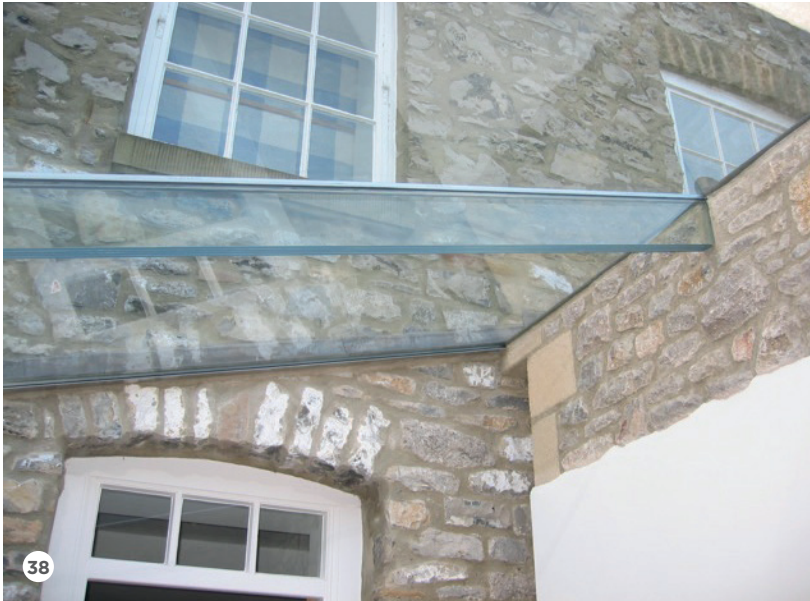
38: This glazed link allowed extension to historic cressbrook mill without harm to the buildings integrity.
