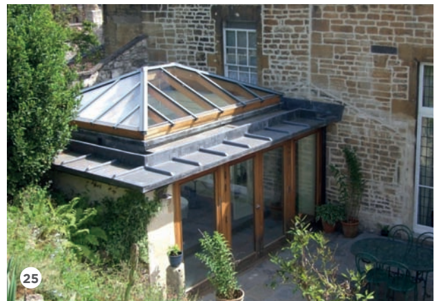
25: A modern extension to the rear of an historic building outside the Park. Note how the roof form allows the first floor window to retain light and view.
