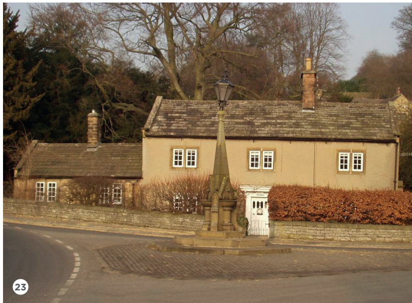
23: A modest, single storey side extension to this listed building in Bakewell allows the original house to retain its dominance and character
