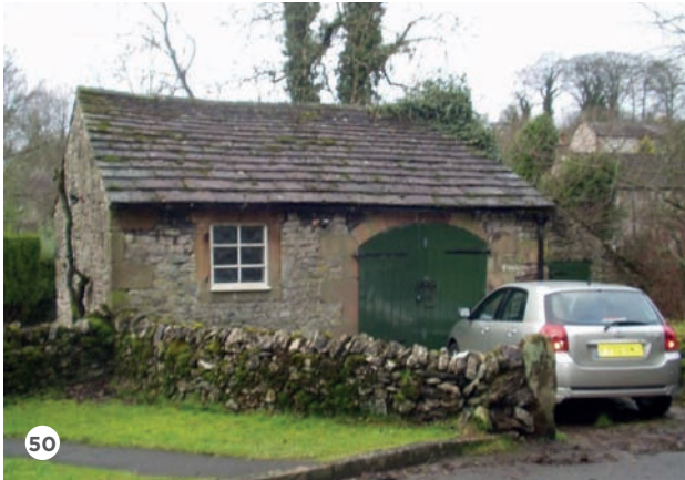
50: Traditional outbuilding in Alport incorporating a cart shed
